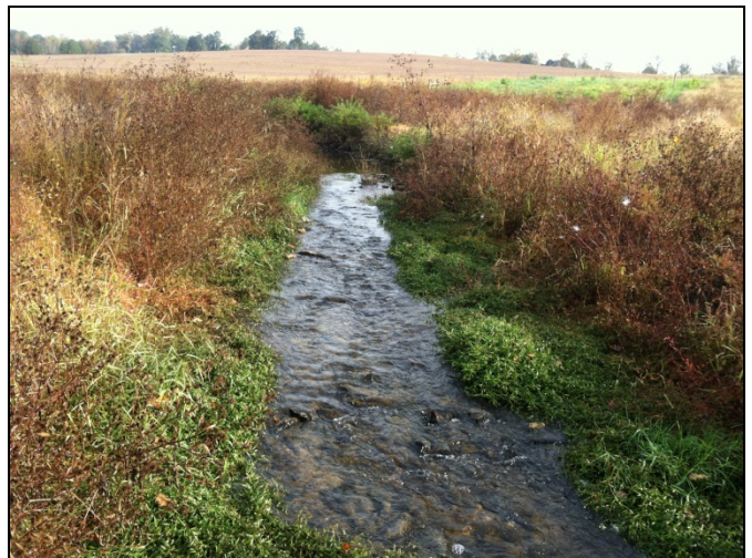
PP 24 STA 46+00, Constructed Riffle
