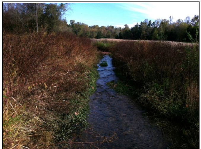
PP 54 STA 24+00, Constructed Riffle
