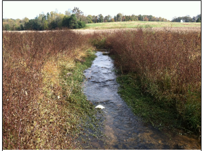
PP 50 STA 26+75, Constructed Riffle
