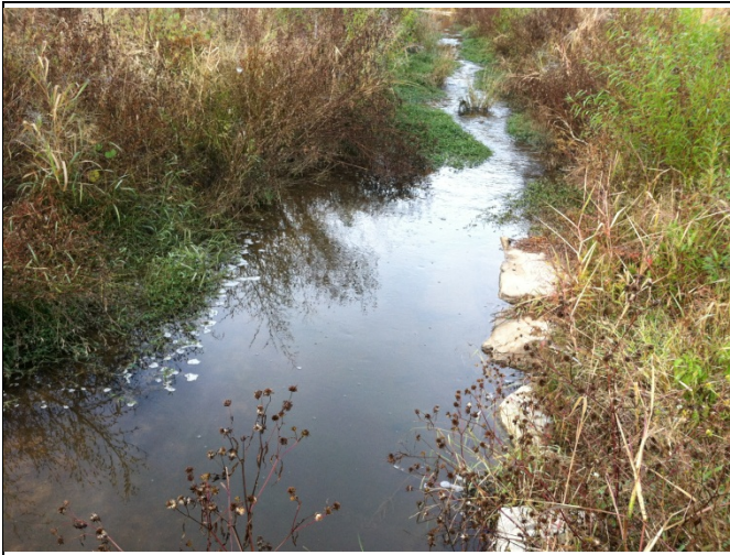
PP 3 STA 60+25, Rock J-Hook
