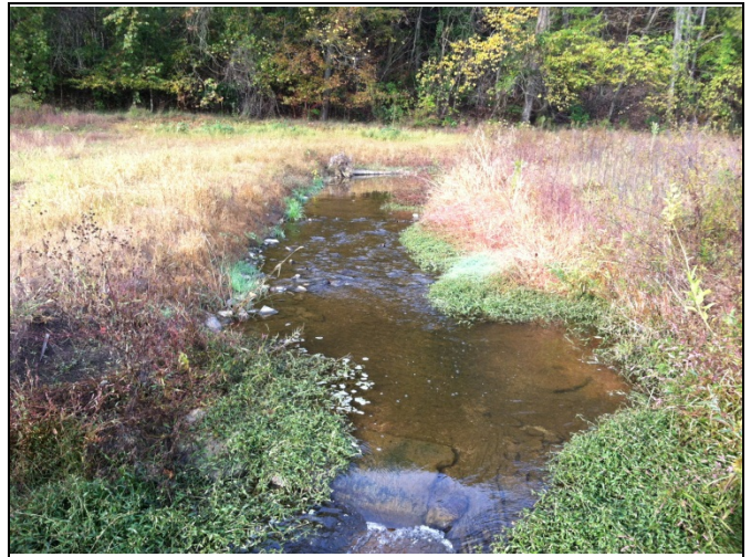
PP 22 STA 47+25, Constructed Riffle
