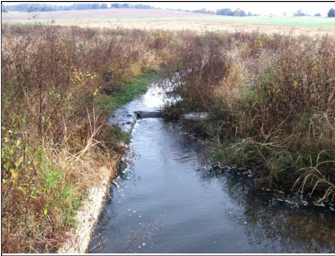
PP 15 STA 52+35, Log J-Hook
