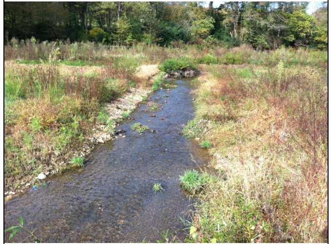
PP 56 STA 22+70, Constructed Riffle
