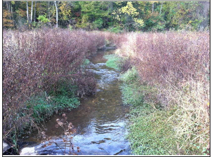
PP 14 STA 53+75, Constructed Riffle
