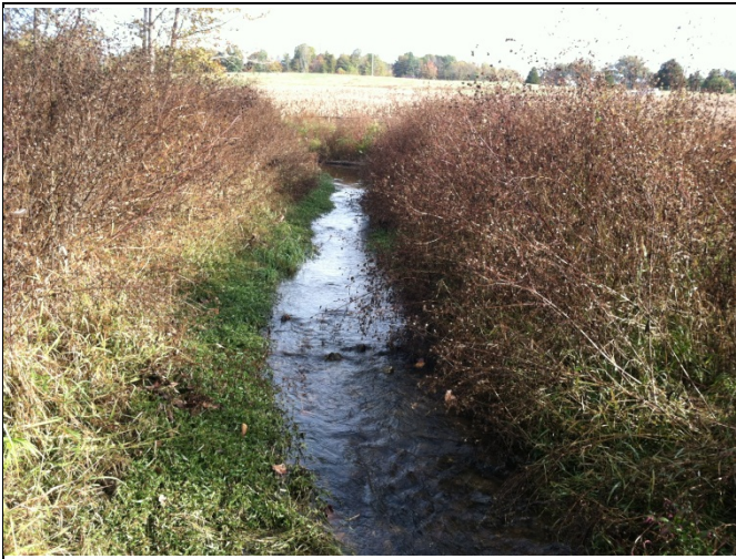
PP 45 STA 30+20, Constructed Riffle
