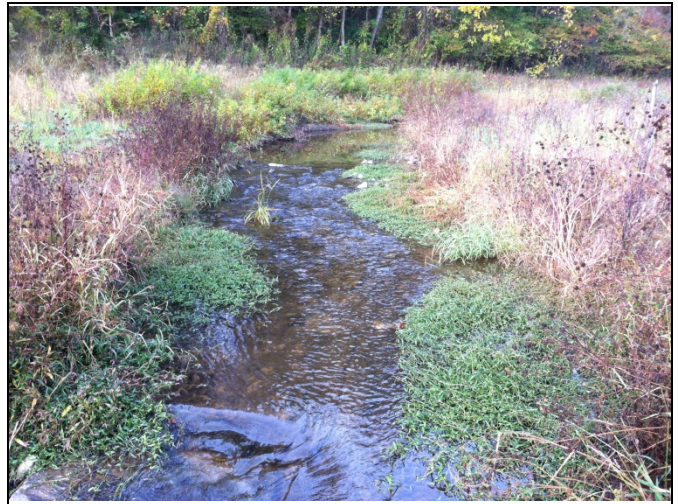
PP 10 STA 56+50, Constructed Riffle
