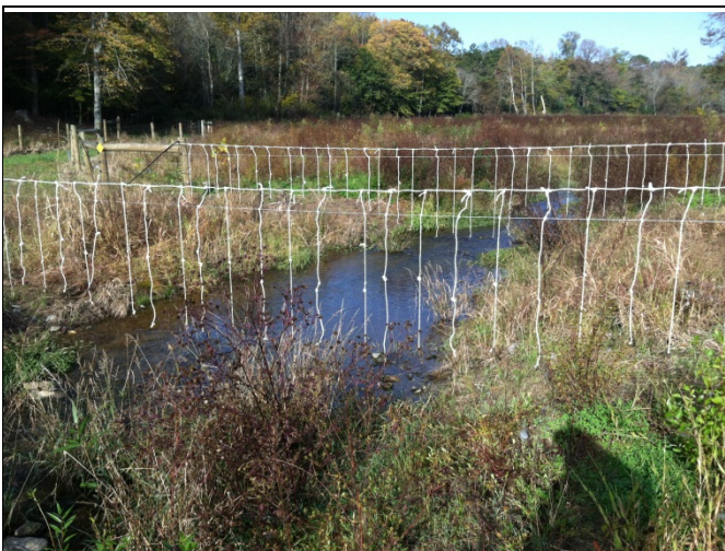
PP 41 STA 33+00, Stream Crossing
