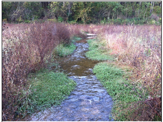
PP 18 STA 50+40, Constructed Riffle
