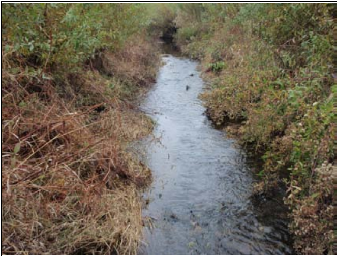
PP 45 STA 30+20, Constructed Riffle
