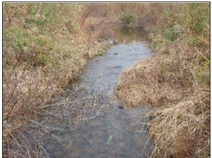
PP 12 STA 55+15, Constructed Riffle
