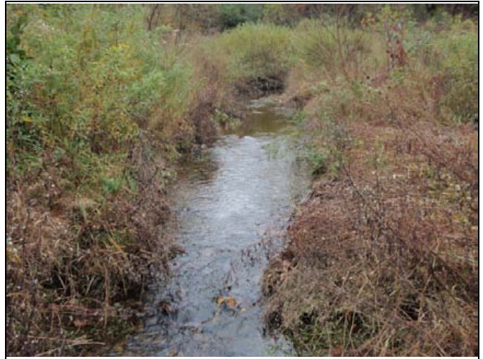
PP 56 STA 22+70, Constructed Riffle
