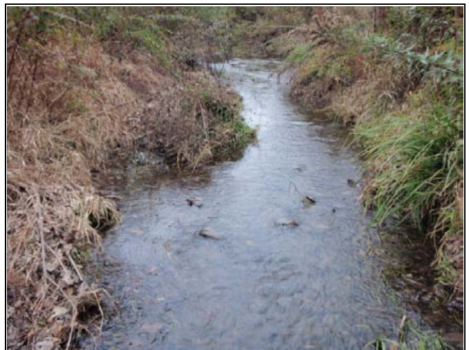
PP 54 STA 24+00, Constructed Riffle
