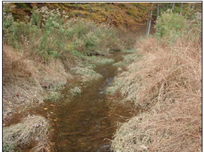
PP 28 STA 43+25, Constructed Riffle
