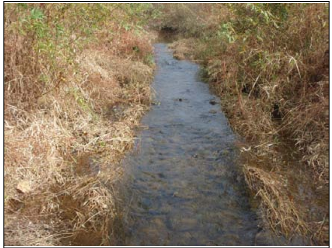
PP 16 STA 52+05, Constructed Riffle
