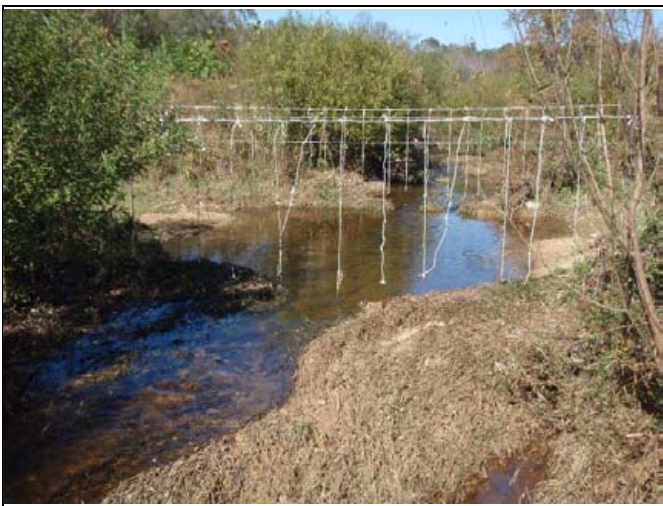
P 41 STA 33+00, Stream Crossing
