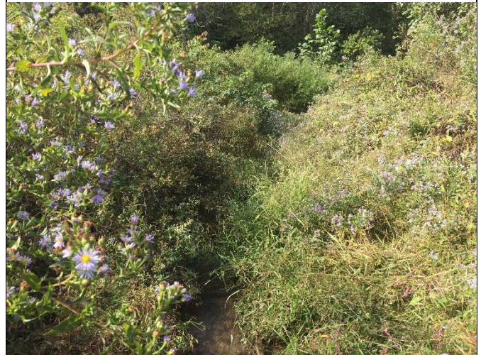
PP 14 STA 53+75, Constructed Riffle
