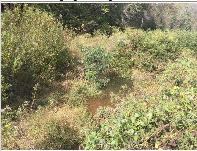
Stream Problem Area 1 - STA 46+50. Bank heavily vegetated. Seems to have stabilized.
