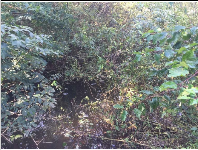
PP 3 STA 60+25, Rock J-Hook
