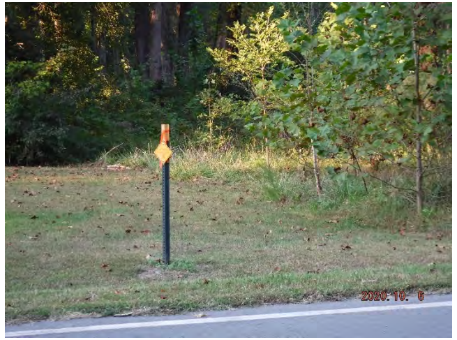
Candy Creek Reach 3 - Easement encroachment at Hopkins Road, LB (Sta. 149+00-150+00) (10/06/2020)
