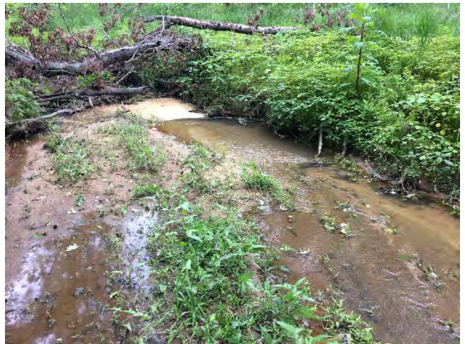
Candy Creek Reach 3 - Aggradation in channel (Sta. 156+10-156+40) (05/13/2020)
