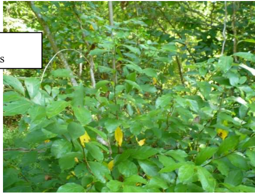
Photos 2-3 Stabilization and staking of left and right banks, respectively, adjacent to ford
