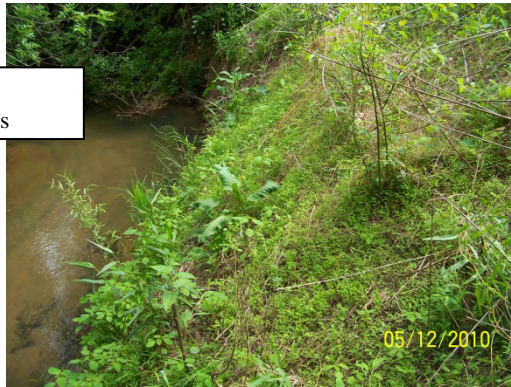
Photos 2-3 Stabilization and staking of left and right banks, respectively, adjacent to ford
