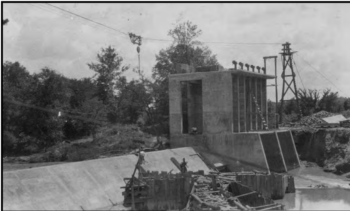
Sandhill Power Company Dam Construction - 1921 (Source: Chatham County Historical Association, 2005)
