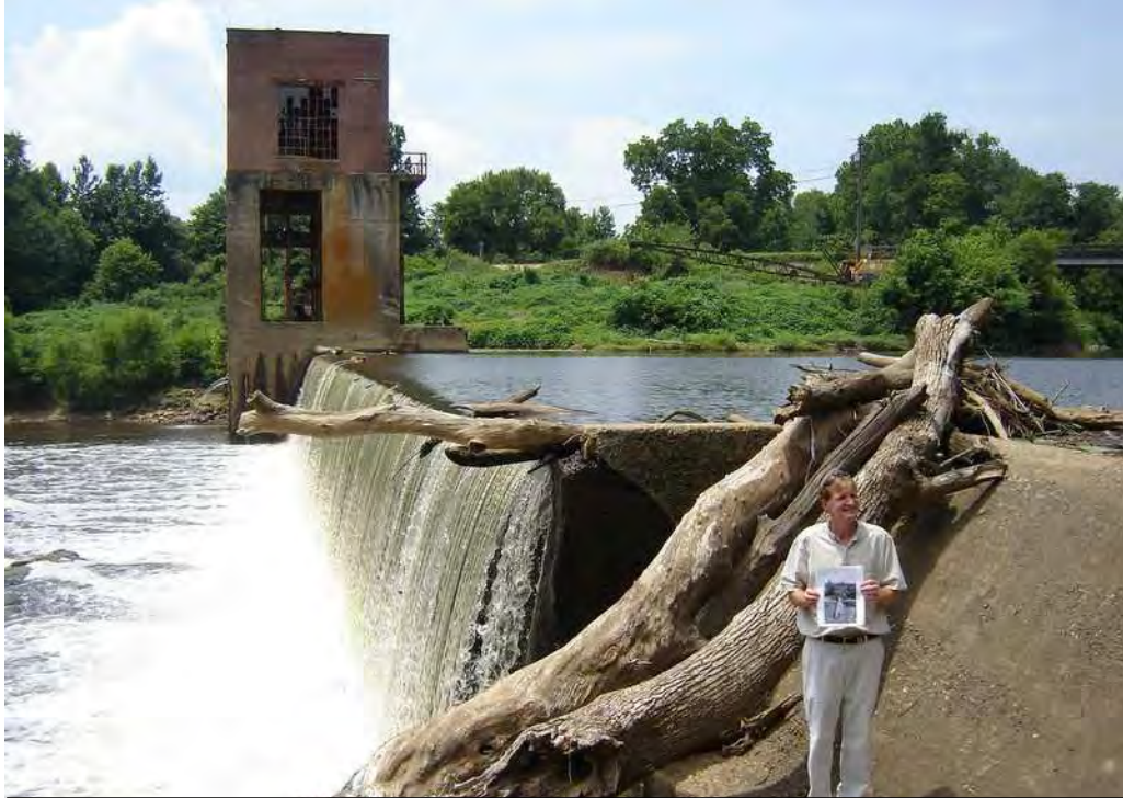
View across ogee and buttressed spillways of the Carbonton Dam. Perspective is from north bank looking south.
