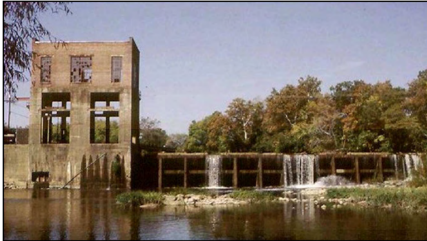
Carbonton Dam Showing Buttresses On Downstream Face (Source: NCDENR-DWR; Instream Flow Web page)
