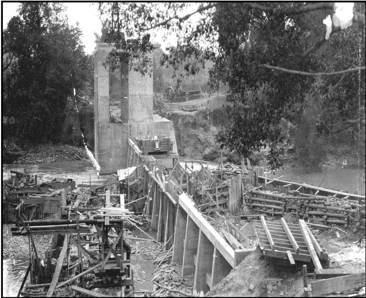
Sandhill Power Company Dam Construction - 1921 (Source: Chatham County Historical Association, 2005)
