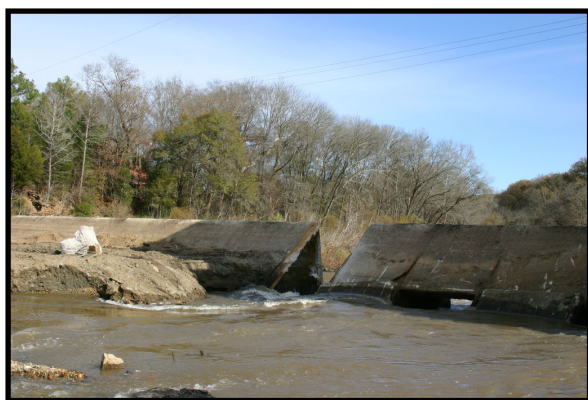
Photos 8 and 9. Constructed notch in cell 1-5 on the southern end of the buttress spillway Source: Restoration Systems 2005
