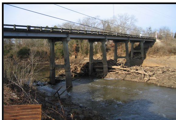
Photo 11. Woody debris island near NC42 bridge dewatering
