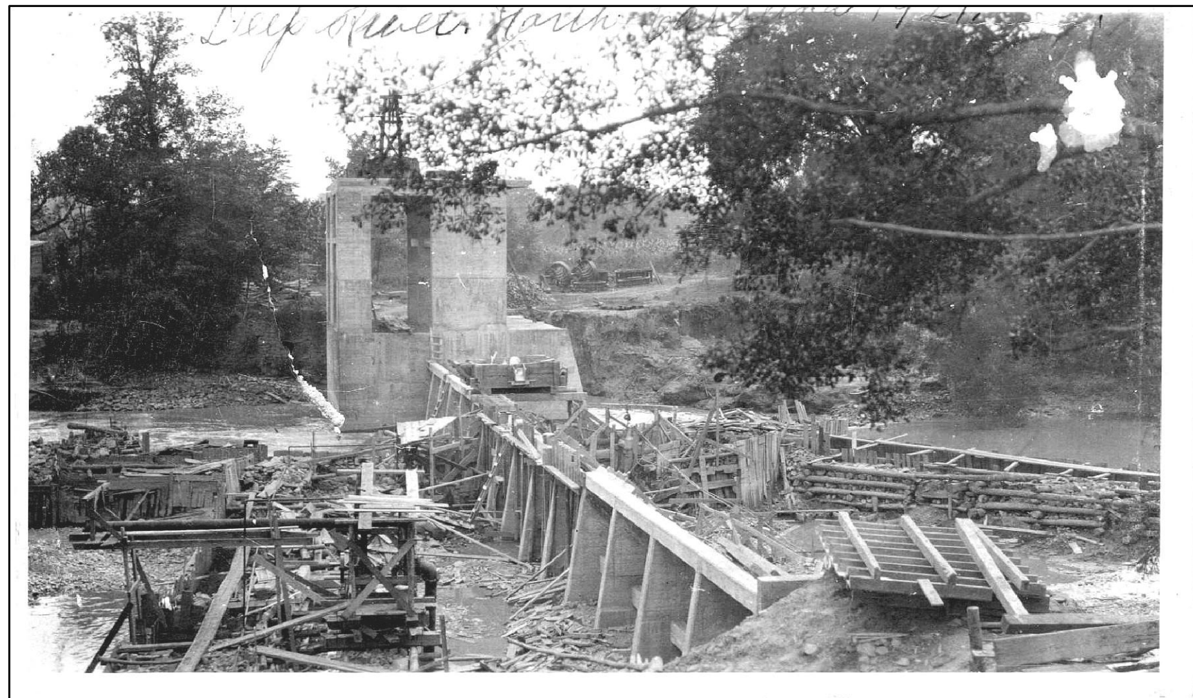
1921 CONSTRUCTION PHOTOGRAPH NOTE THAT OGEE SPILLWAY IS NOT YET CONSTRUCTED
