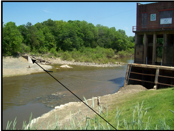
Photo 16. After dam removal, the ogee spillway was retained
