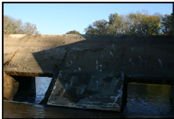
Photo 7. Dewatering through mud gates on dam spillway
