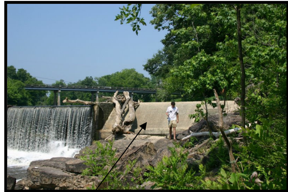
Photo 17/ Ogee spillway in pre-removal photo
