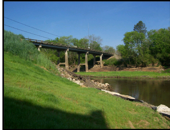
Photo 15. Regraded southern bank of the Deep River behind the powerhouse. Slope was revegetated
