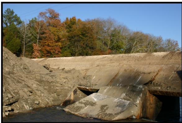
Photo 6. Uncovered mud gates on dam spillway
