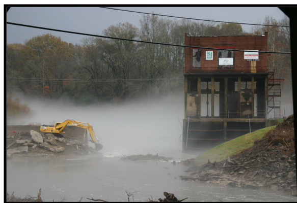
Photos 8 and 9. Constructed notch in cell 1-5 on the southern end of the buttress spillway Source: Restoration Systems 2005
