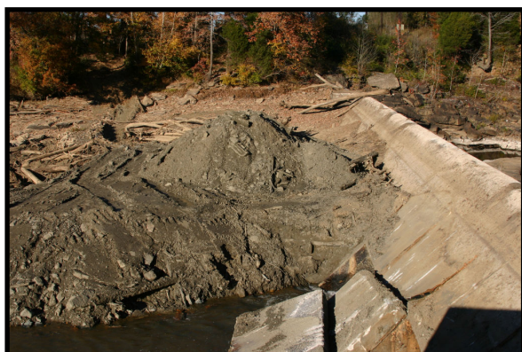
Photo 10. Substrate behind dam spillway after
