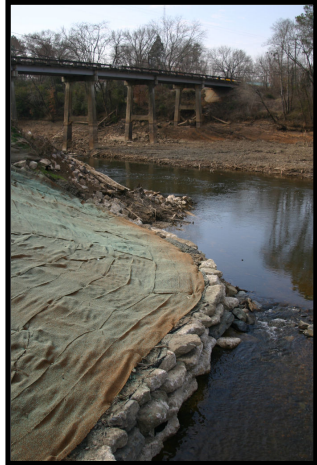
Photo 14. Bank toe protection created from dam spillway debris
