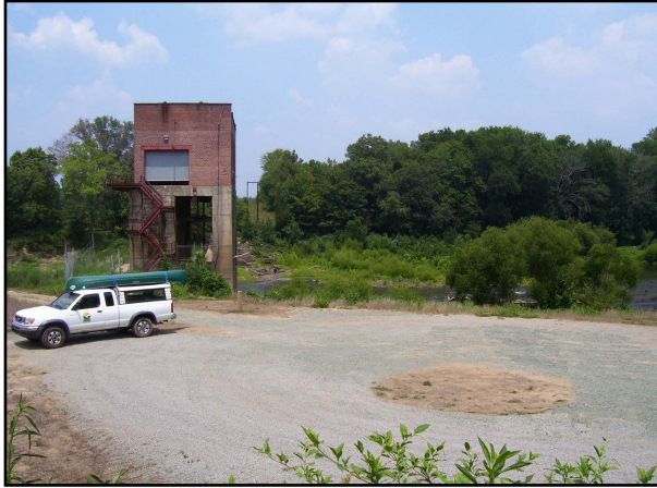
Boat launch adjacent to historic powerhouse, Deep River Park
