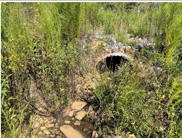
PHOTO POINT 4A - Carpenter Bottom R1 - upstream (8/31/2022)
