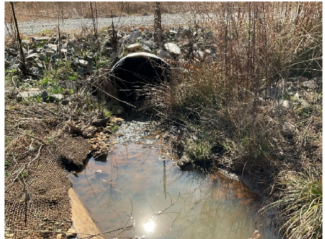
PHOTO POINT 4 - Carpenter Bottom R1 - downstream (03/06/2023)
