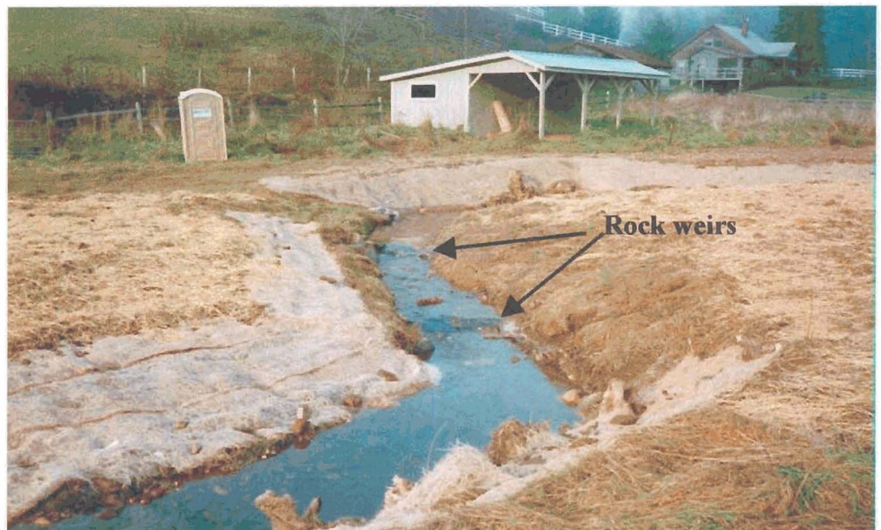
Riffle section between second and third meander, station 2+46 to 1+59.
