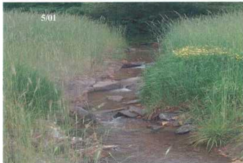
FIGURE A2.2.—Upper end of channel showing stable step pools, looking upstream from station +82 to +92.
