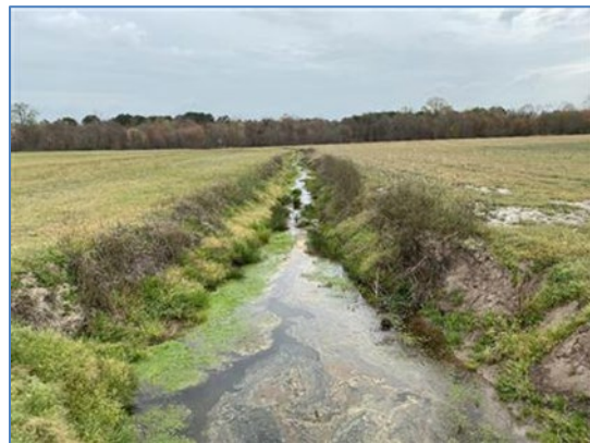
Looking Downstream along BH1 March 23, 2022
