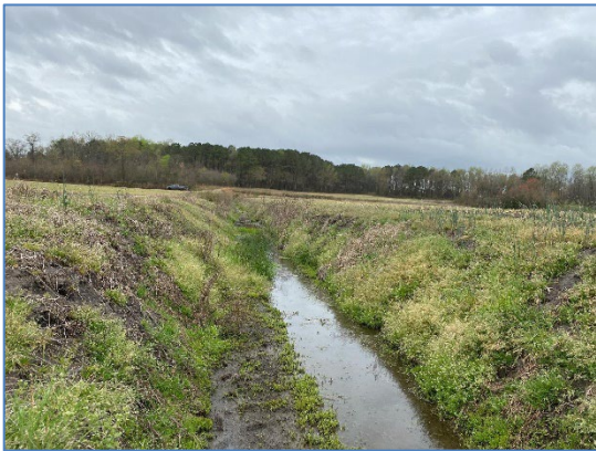
Looking Upstream along BH3 March 23, 2022
