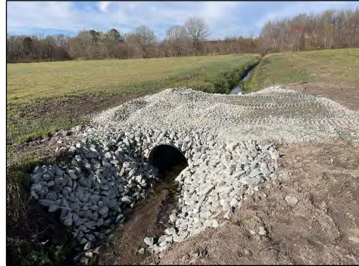
Culvert installation (2/28/2023)
