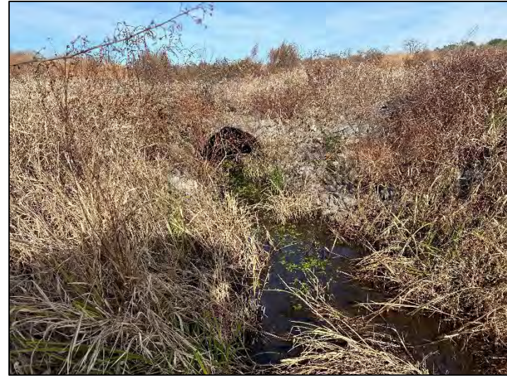
BH3 Culvert Upstream (12/13/2023)
