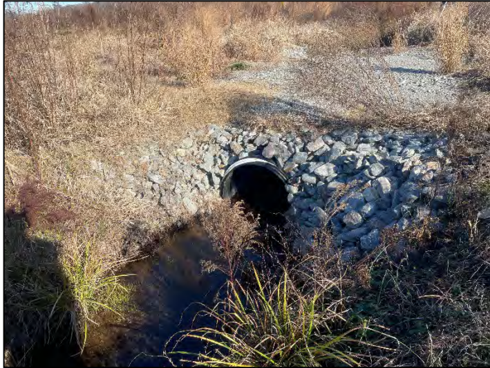
BH1 Culvert Downstream (12/12/2023)
