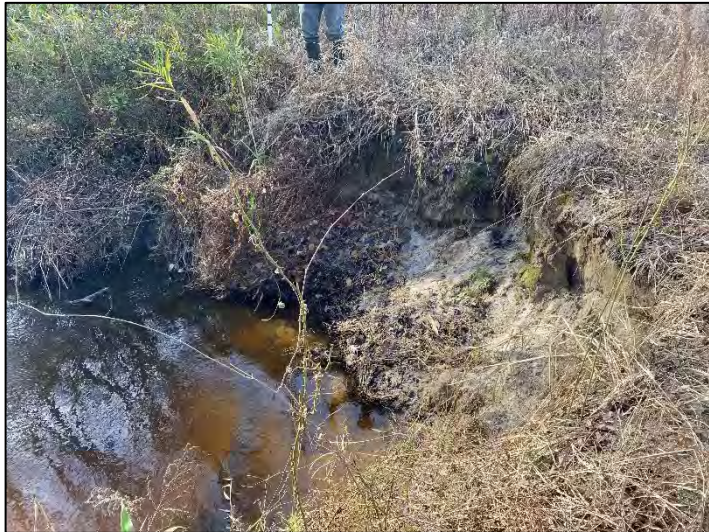
Left Bank Erosion Carraway Creek (12/13/2023)
