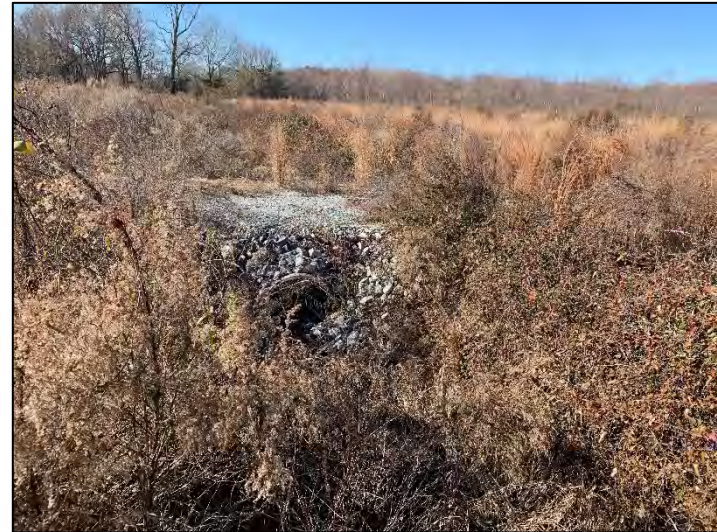
BH2 Culvert Upstream (12/12/2023)
