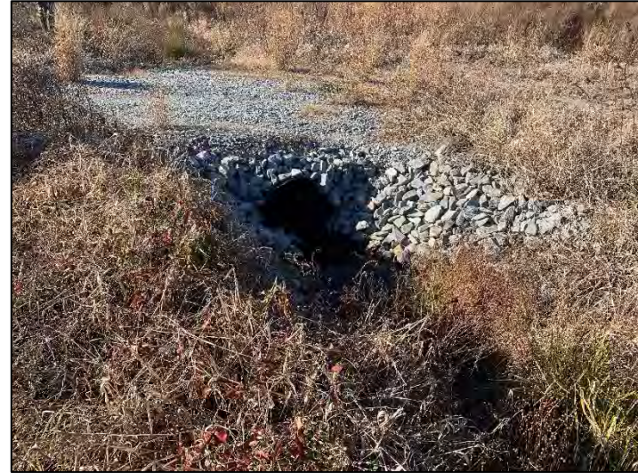
BH1 Culvert Upstream (12/12/2023)
