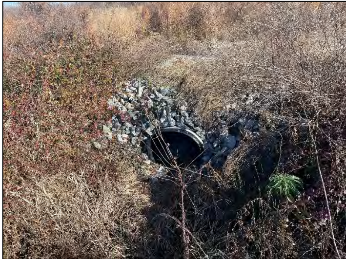
BH2 Culvert Downstream (12/13/2023)
