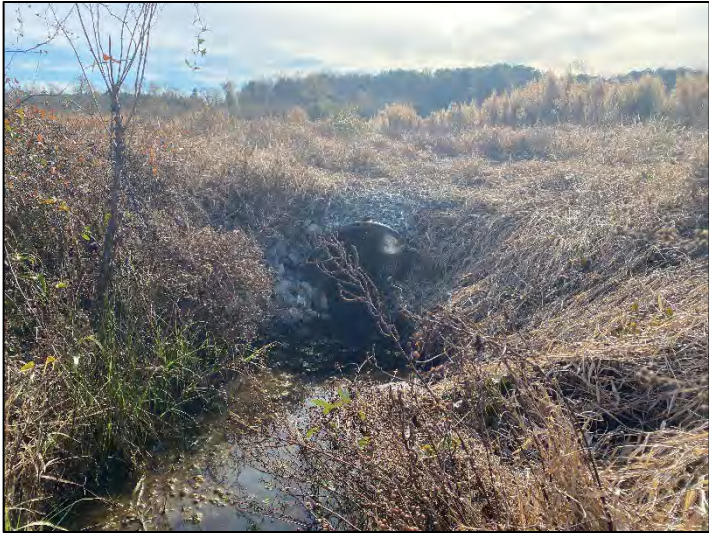
BH3 Culvert Downstream (12/13/2023)
