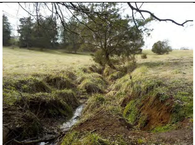
DS1 – Looking Upstream (2/1/2018)
