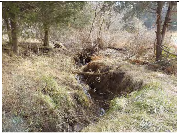
DS1 – Looking Upstream (2/1/2018)
