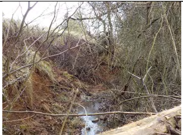
DS1 – Looking Downstream (2/1/2018)
