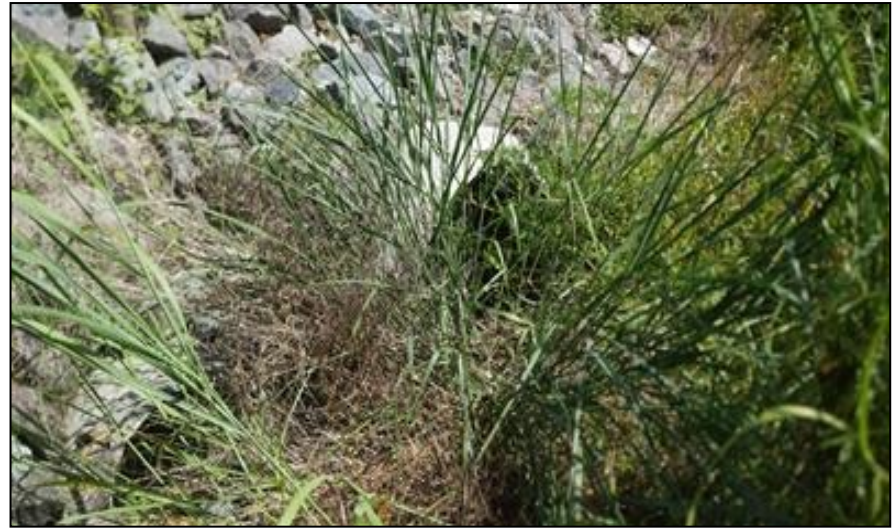
Culvert DS1 Downstream (10/5/2022)
