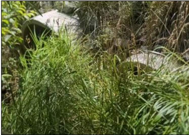
Culvert DS1 Upstream (10/05/2022)
