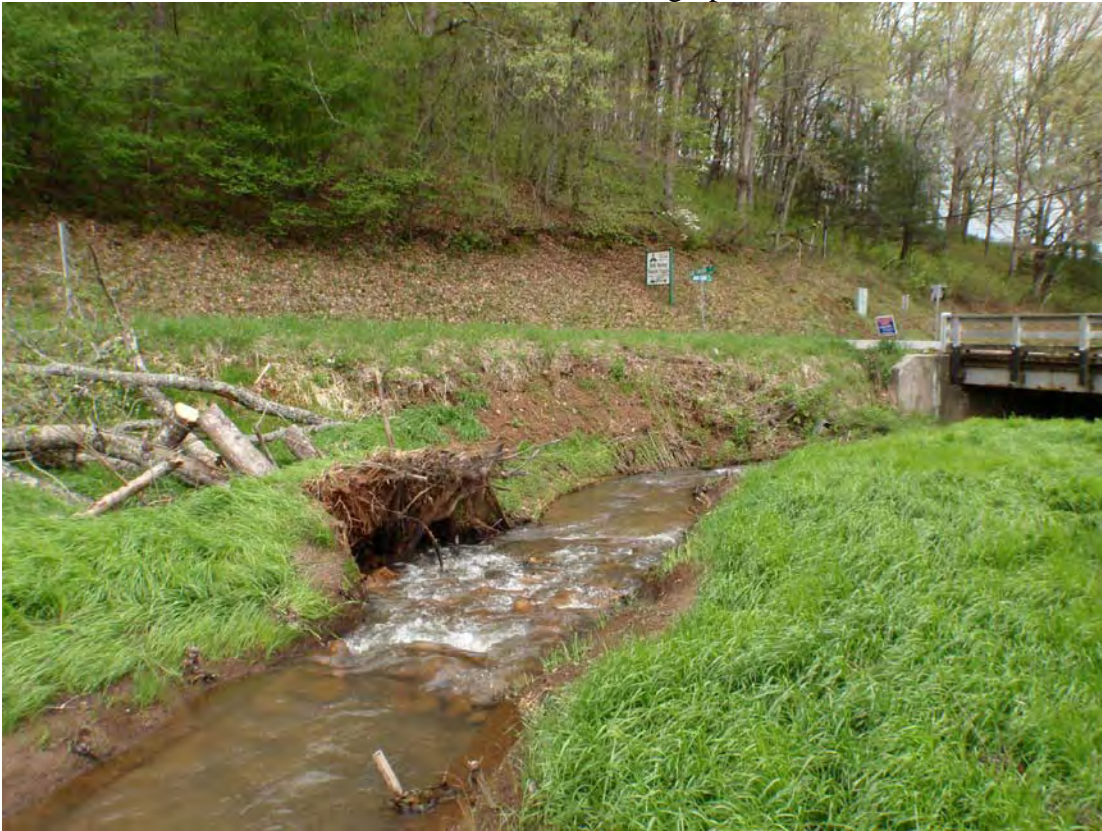
Stream Station 3 – 6/11/2010 – Year 1 Monitoring
