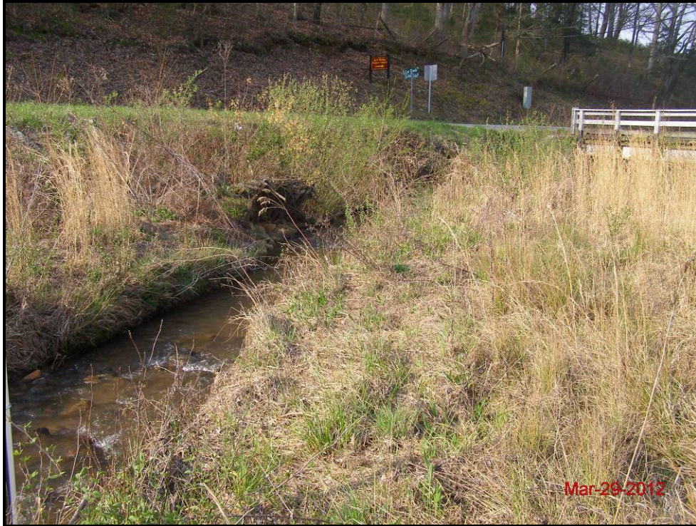
Cat Creek – Permanent Photo Station 3 Station 15+98 - Downstream
