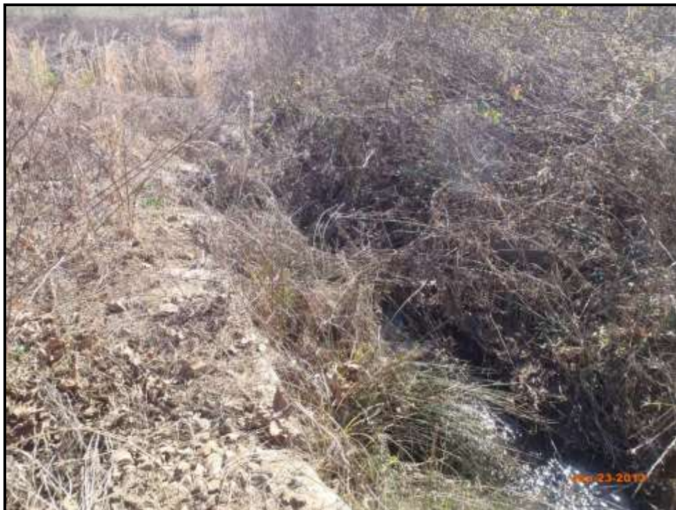
UT4 – Permanent Photo Station 8 Station 402+08 - Upstream
