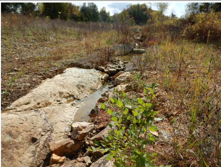
PHOTO POINT 15 UT1 R3 – upstream (10/22/2020)
