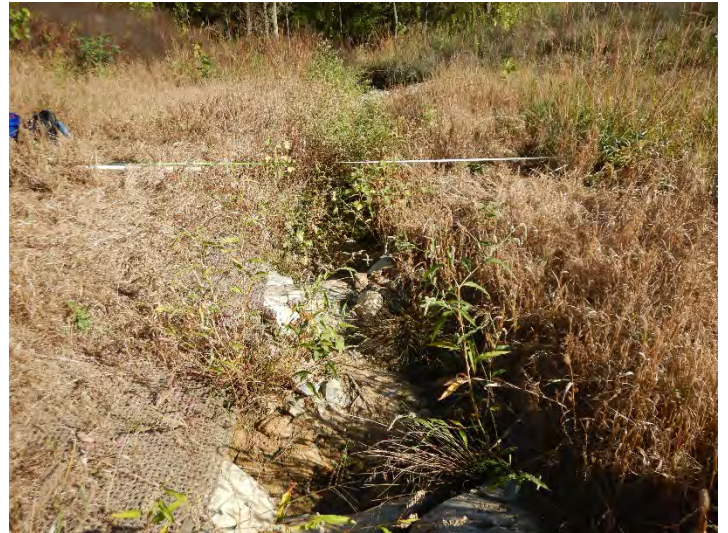
UT1 R3 XS7 downstream – Area of Bedload Movement (Post-Repair) (10/18/2021)
