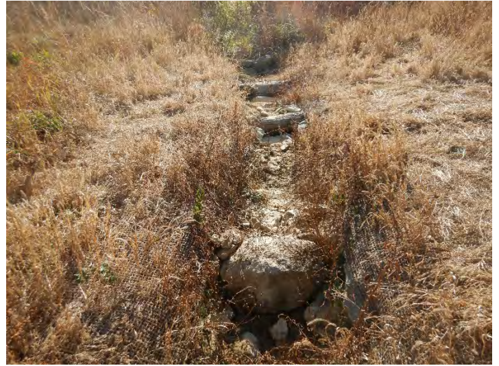
UT1 R3 upstream – Area of Bedload Movement (Post-Repair) (11/18/2021)
