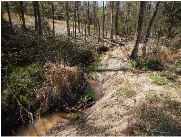
PHOTO POINT 10 UT1 R1 – upstream (04/02/2021)
