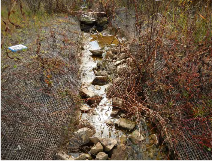
UT1 R3 upstream – Area of Bedload Movement (Pre-Repair) (10/22/2020)
