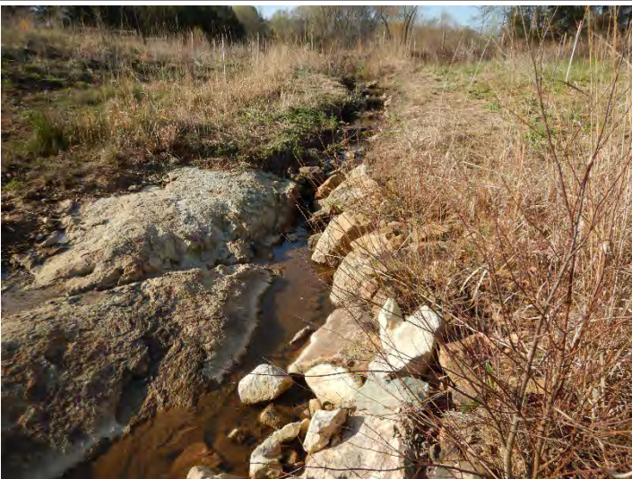
PHOTO POINT 15 UT1 R3 – upstream (04/05/2022)
