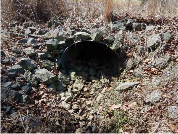
Catfish Creek R4 – Looking Upstream (03/14/2023)
