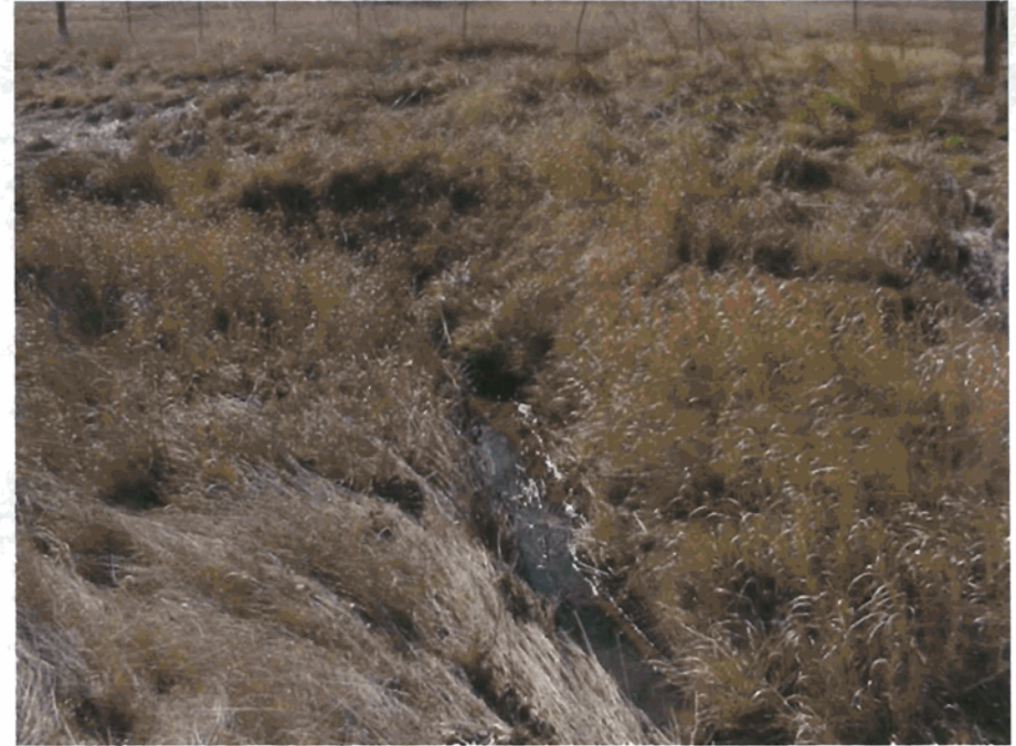
Photo Station 17.A: Looking downstream of culvert outlet.
