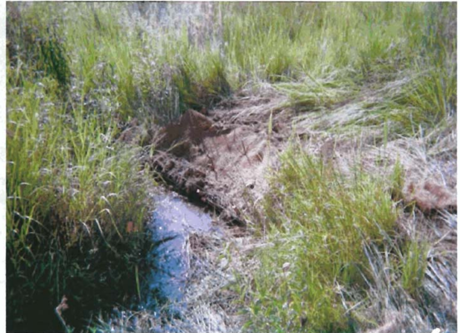
Photo 2: Looking at erosion fix between Stations 20+00 and 20+50
