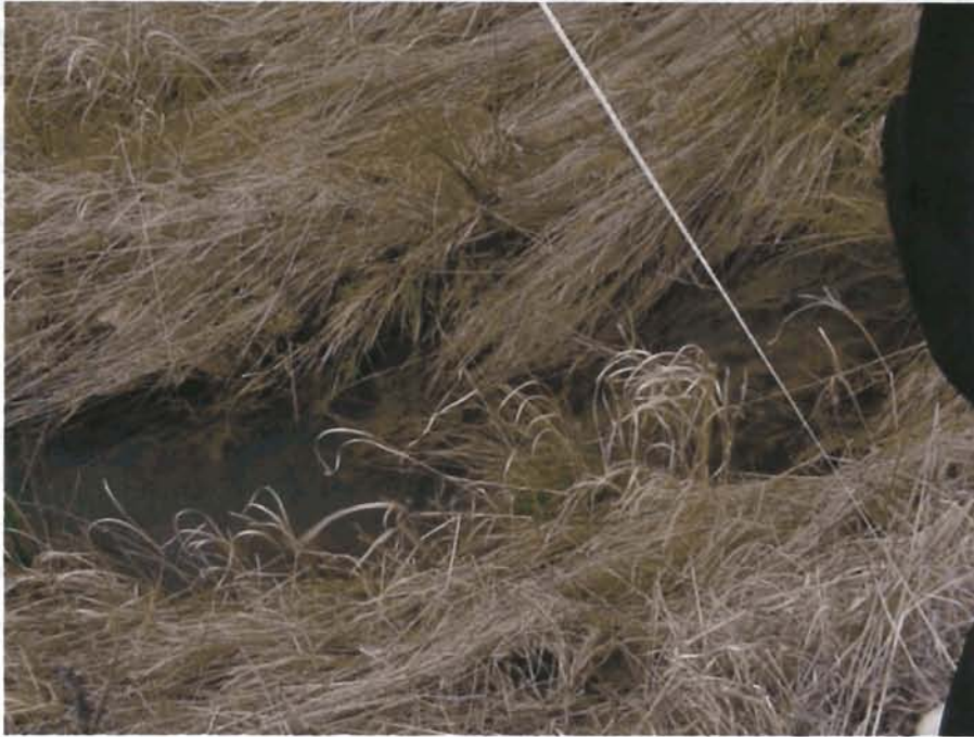
Photo Station 12.A: Looking at cross-section 5.
