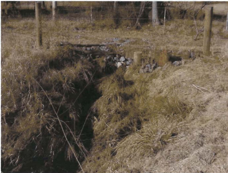
Photo Station 17.B: Looking upstream at culvert face.
