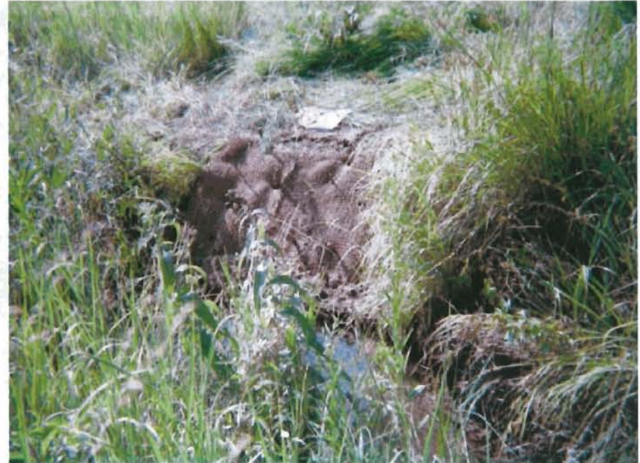
Photo 4: Looking at erosion fix on outer bend downstream of Station 20+00
