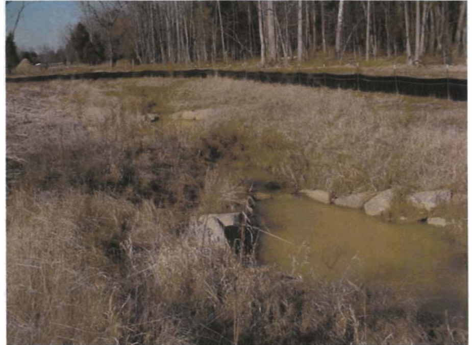
Photo Station 3.B: Looking upstream at cross vanes 7 and 8.
