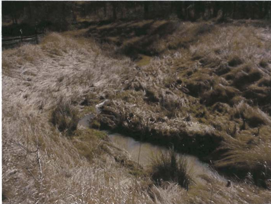
Photo Station 2.A: Looking downstream at cross vanes 3 and 4.
