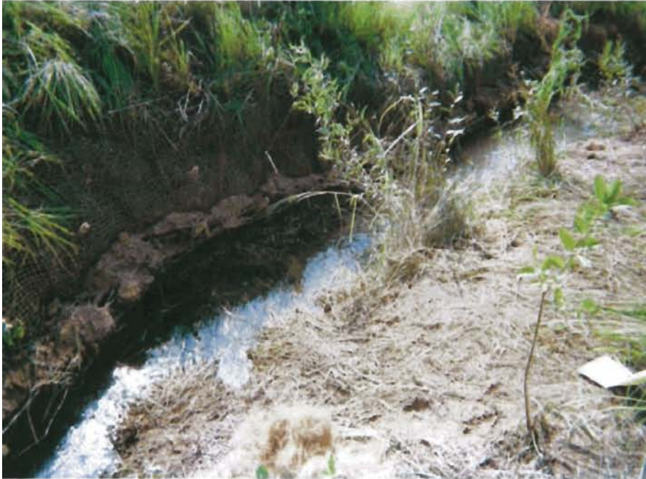
Photo 3: Looking at erosion fix between Stations 20+20 and 20+50
