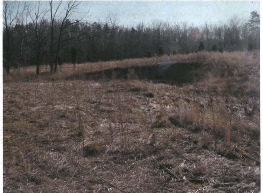
Photo Station 6.A: Looking downstream at right bank.
