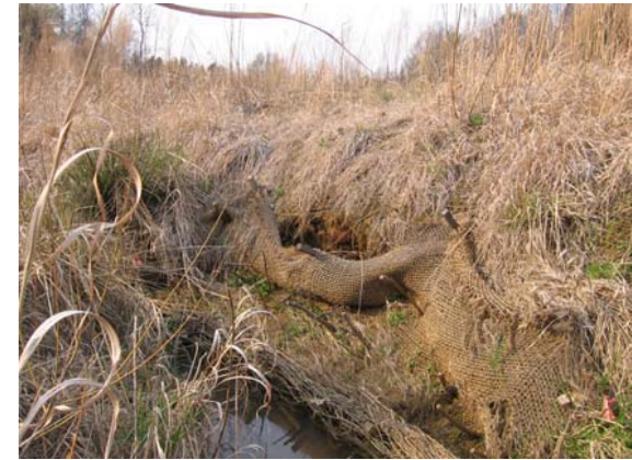
2. Bank Erosion: Severe – 3/30/06
