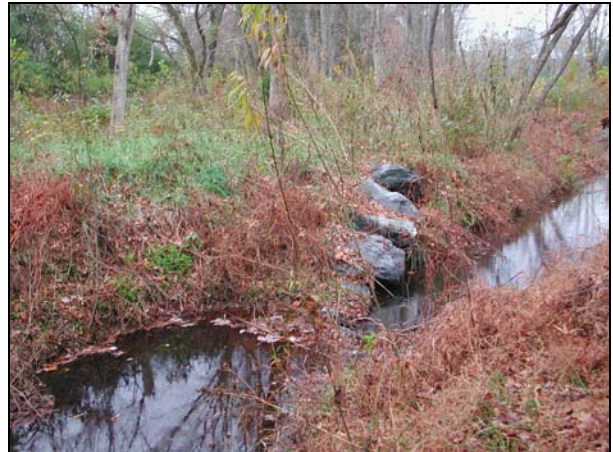
Sta. 24+15 Tibbs Run DS at J-hook vane and pool
