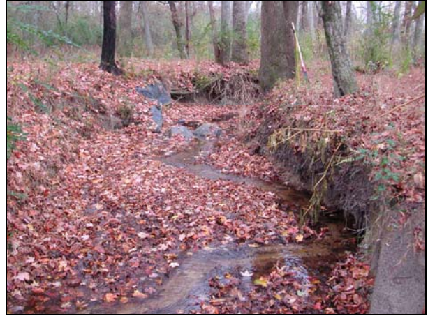
Sta. 27+00 Tibbs Run DS at J-hook vane and pool
