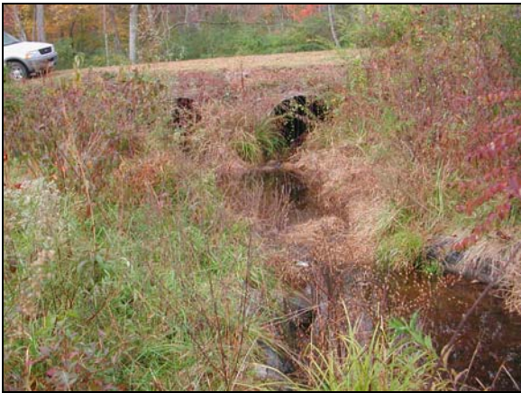
Sta. 57+50 West Branch US at X-vane
