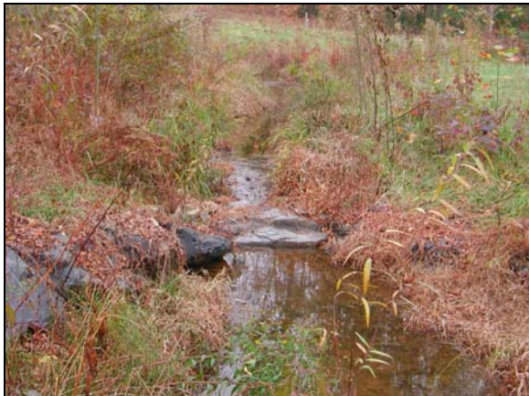
Sta. 50+80 West Branch US at X-vane with rock seal
