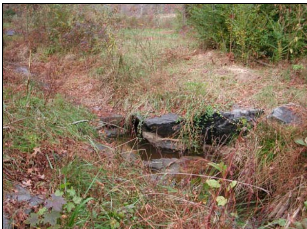
Sta. 14+34 West Branch US at X-vane with rock seal
