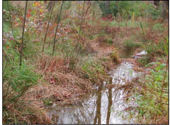
Sta. 51+50 West Branch DS at X-vane and Test Plot #1
