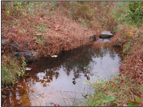
Sta. 17+10 Tibbs Run US at J-hook vane and pool
