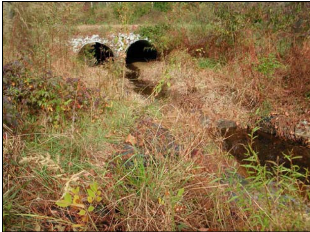
Sta. 12+50 Tibbs Run US at X-vane and pipe crossing
