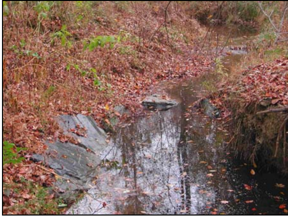
Sta. 30+90 Tibbs Run US at J-hook vane and pool
