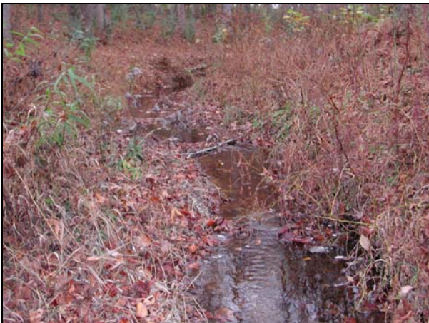
Sta. 25+60 Tibbs Run US at run prior to X-vane
