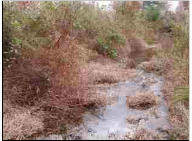
Sta. 11+10 Tibbs Run Downstream (DS) at riffle, X-vane, and culvert
