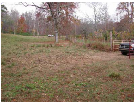
SPA5. Station 53+50. Poor drainage because of improper grading. Picture taken during severe drought.
