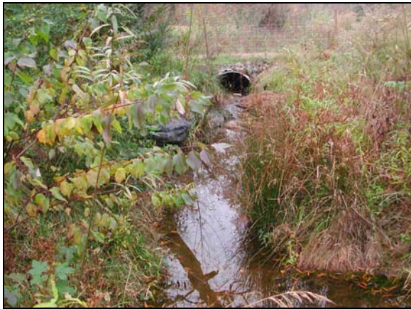
Sta. 53+00 West Branch US at X-vane and pipe crossing
