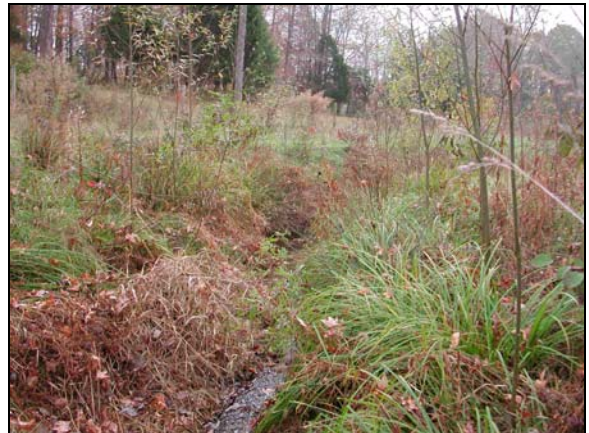
Sta. 55+40 West Branch DS at log vanes
