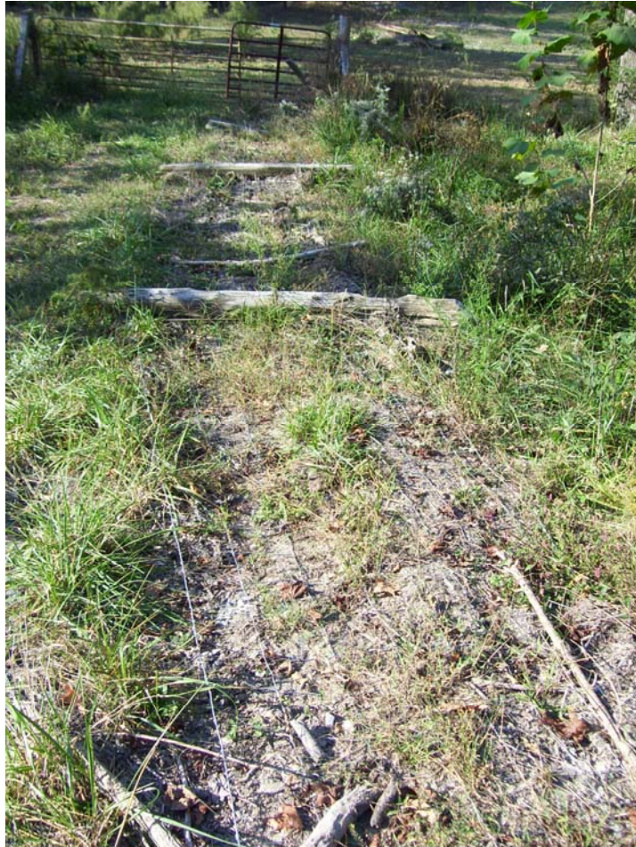
SPA 1. Damaged fence.
