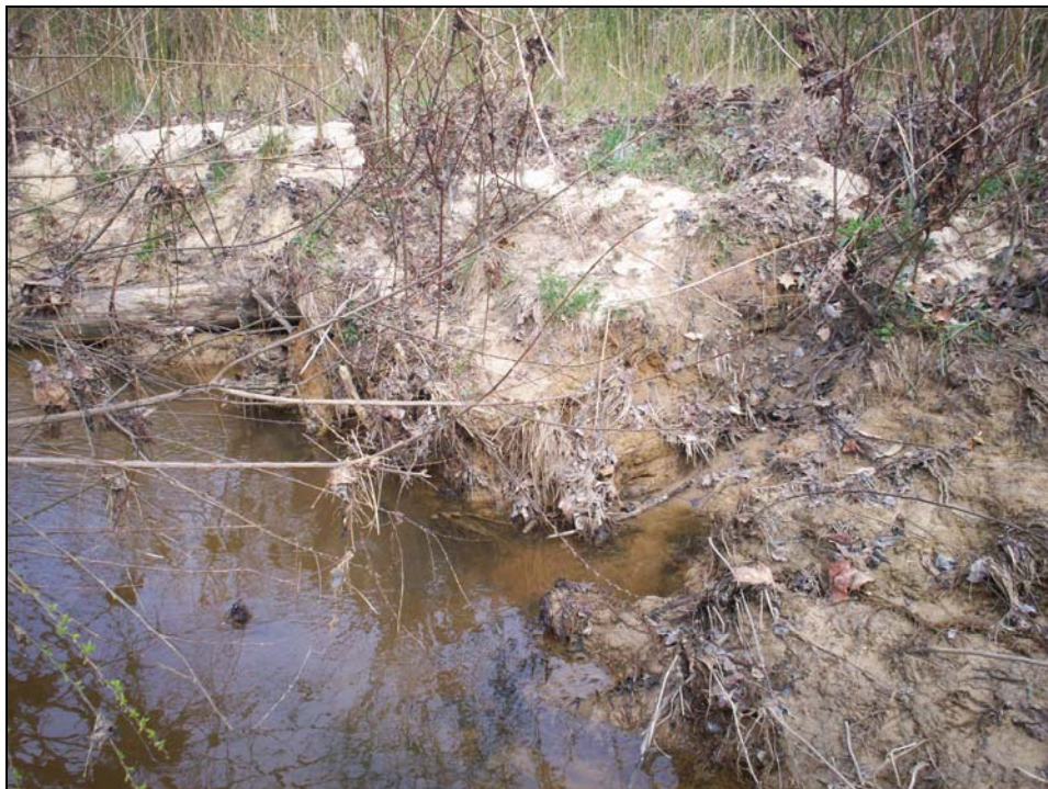
SPA 7. Bank failure behind log vane.
