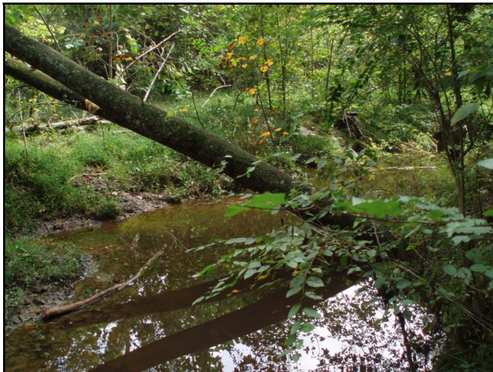
PA #8 – Bank erosion/tree falling across channel. Sta. 24+25
