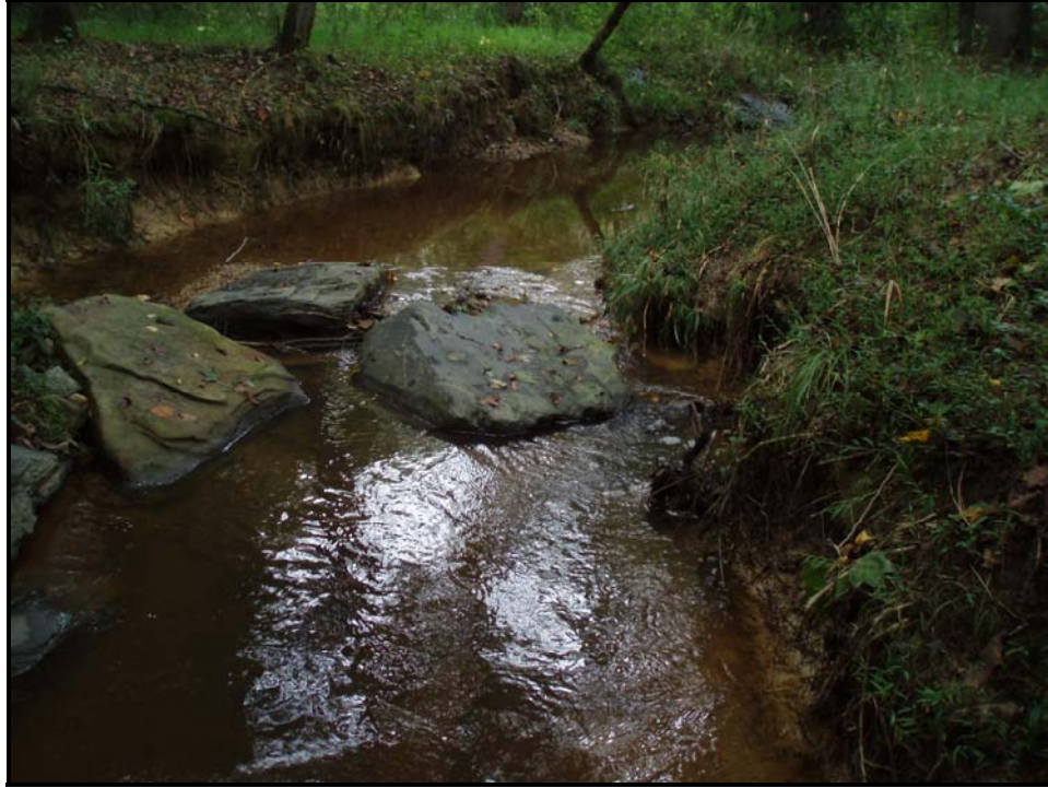
PA #17 – Erosion at cross vane. Sta. 30+80
