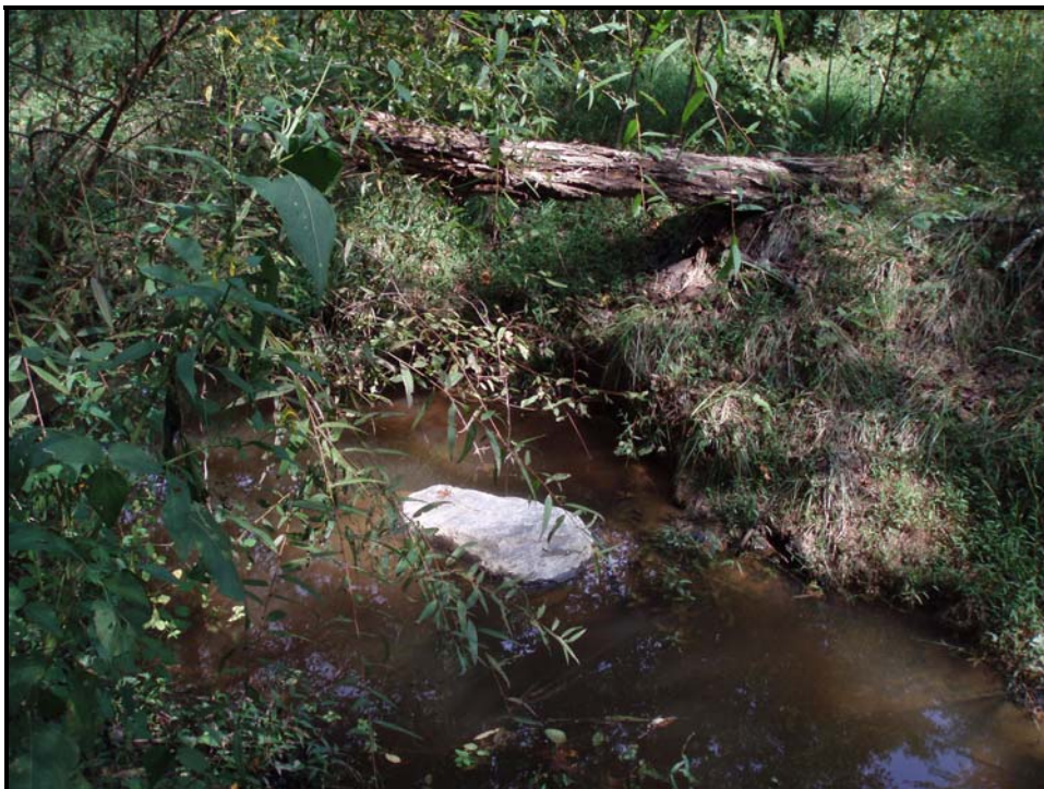
PA #10 – Left bank erosion at cross vane. Sta. 25+60
