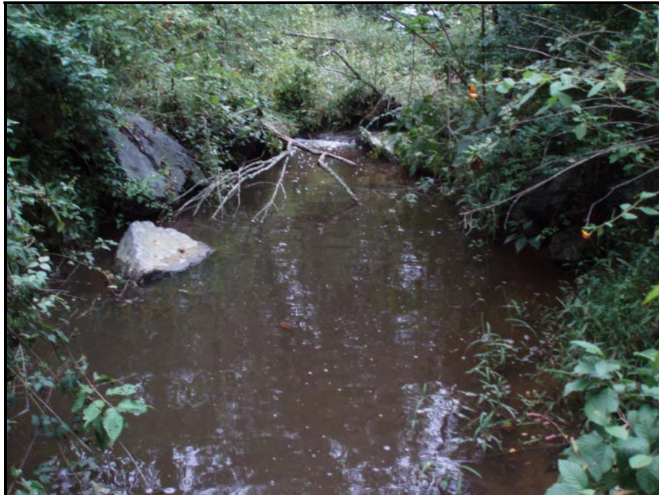
PA #18 – Bank failure at cross vane. Sta. 32+00
