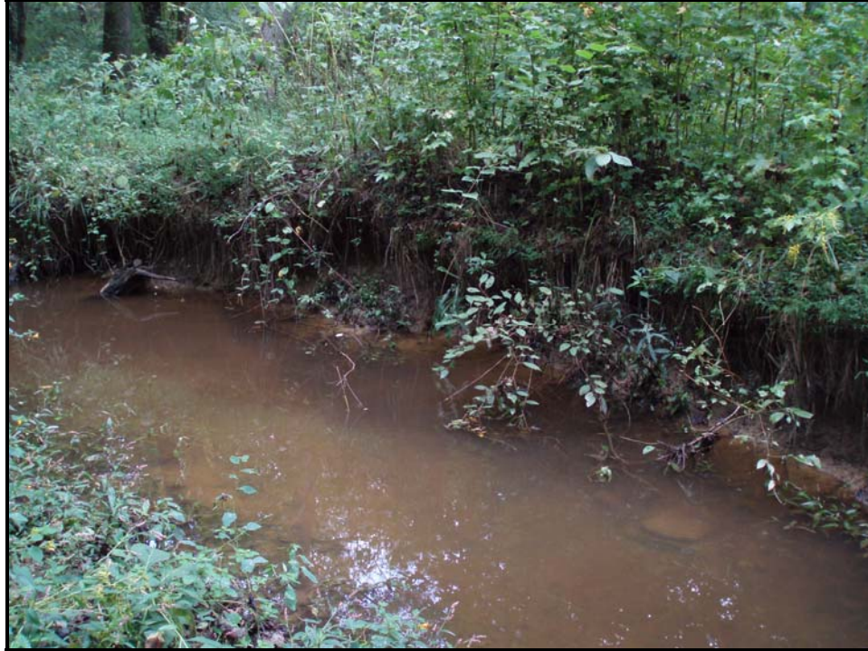
PA #11 – Left bank erosion/undercut bank. Sta. 26+50 to 27+00
