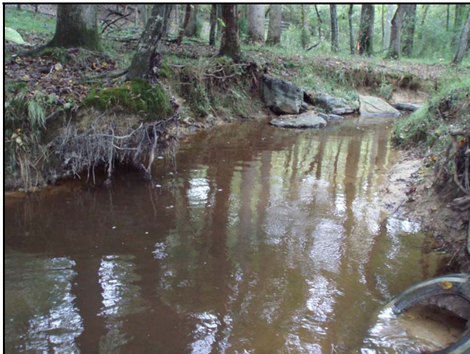
PA #16 – Right bank undercut. Sta. 30+50
