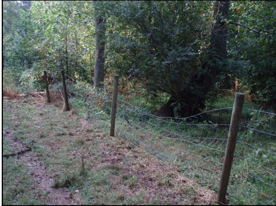
PA #5 – Damaged fence. Sta. 14+00
