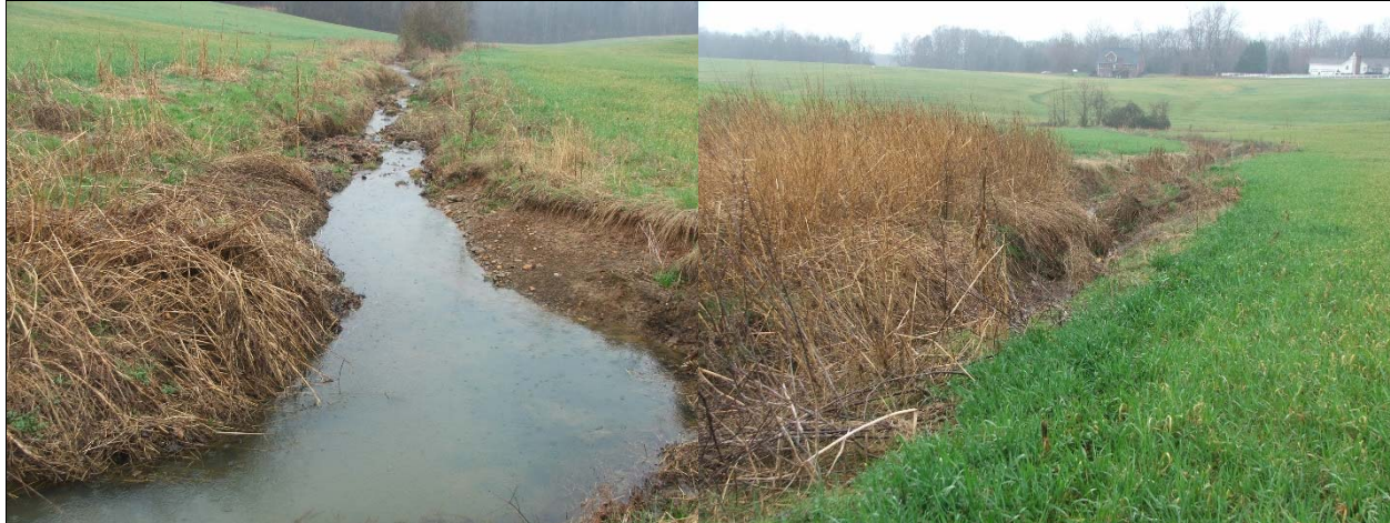
View south and downstream on UTCC. Natural meanders will be returned to the channel and a vegetative buffer will be installed to reduce sediment and nutrient loading. 3/19/15
