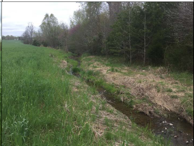
Looking north and upstream at the lower portion of UTCC that is to be relocated. 4/13/15
