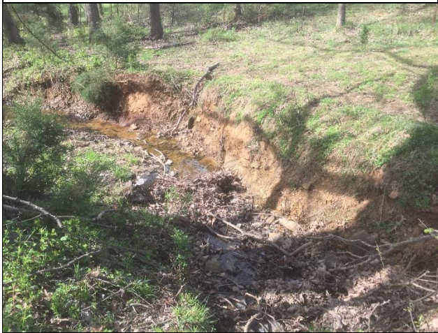
View north and upstream on UTCC. Restoration will integrate the stream with its floodplain. 4/13/15
