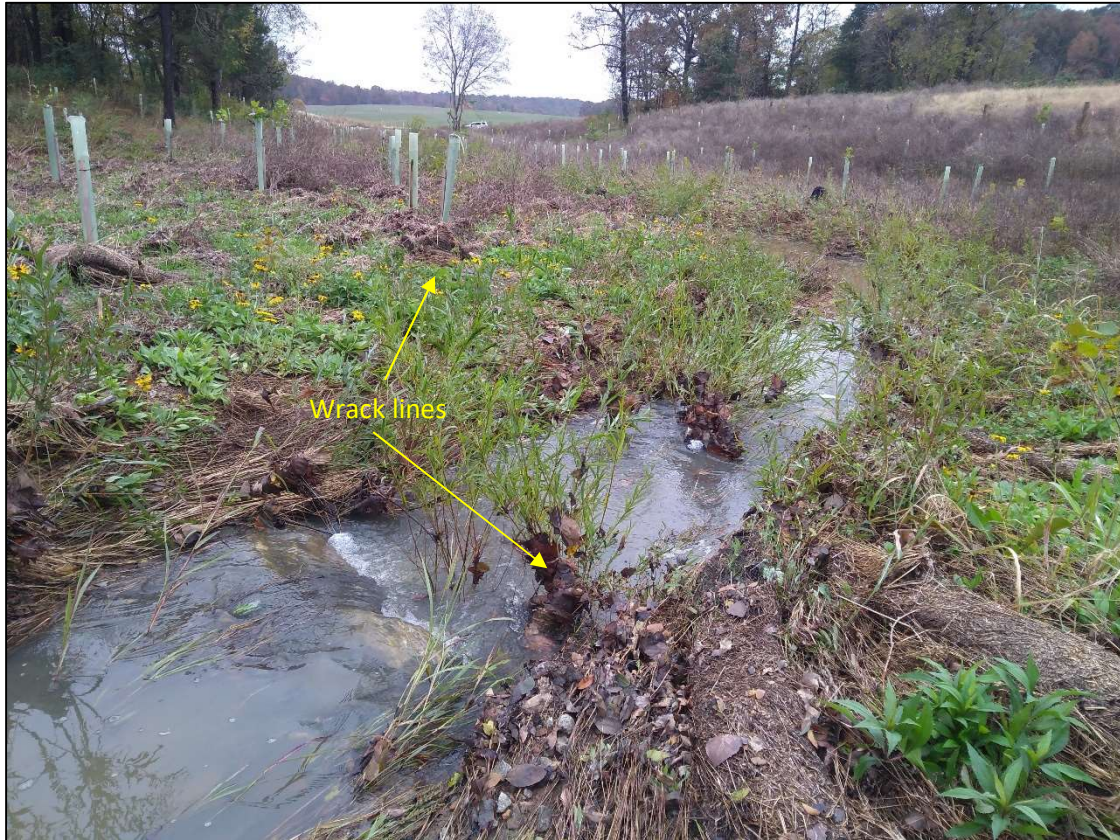
Photo 1. Wrack lines above bankfull, 11/5/2018
