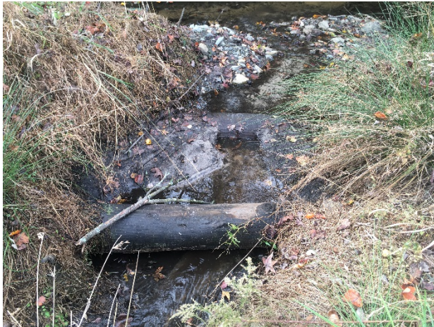
SPA3 – Undercut Log Sills – UT3 @ Sta. 20+10 to 20+00
