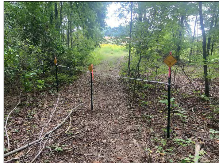
Installed additional easement markers (9/21/2023)
