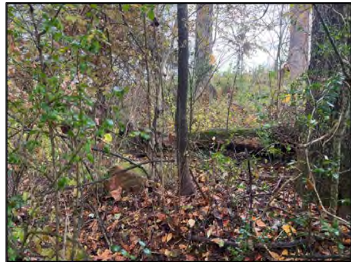
Old Fence Removed (10/31/2023)
