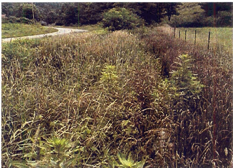
Looking upstream from power pole, showing sloping, erosion controls, vegetation and fencing. Top photo shows reach before construction, middle photo shows constructed channel and lower photo shows the same site 10 months after construction.
