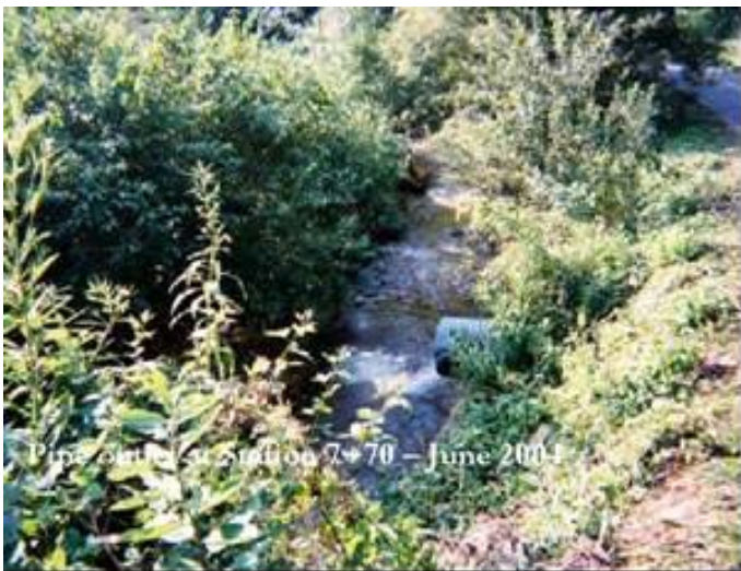
Photo sta. 7+70, looking downstream, June 2004.
