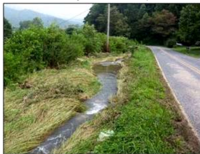
Photo sta. 2+21 looking downstream, August 2004
