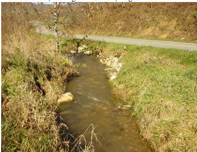
Photo sta. 5+99, looking downstream, November 2003.
