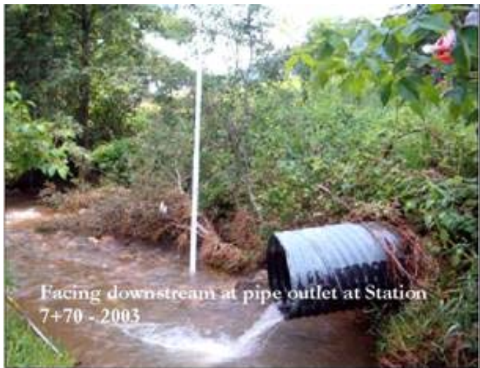
Photo sta. 7+70, looking downstream, July 2003.
