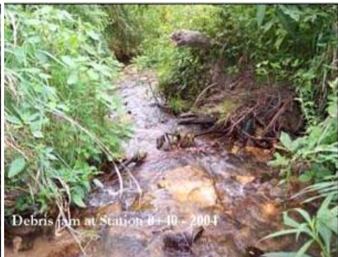
Photo sta. 0+40, looking downstream, June 2004.
