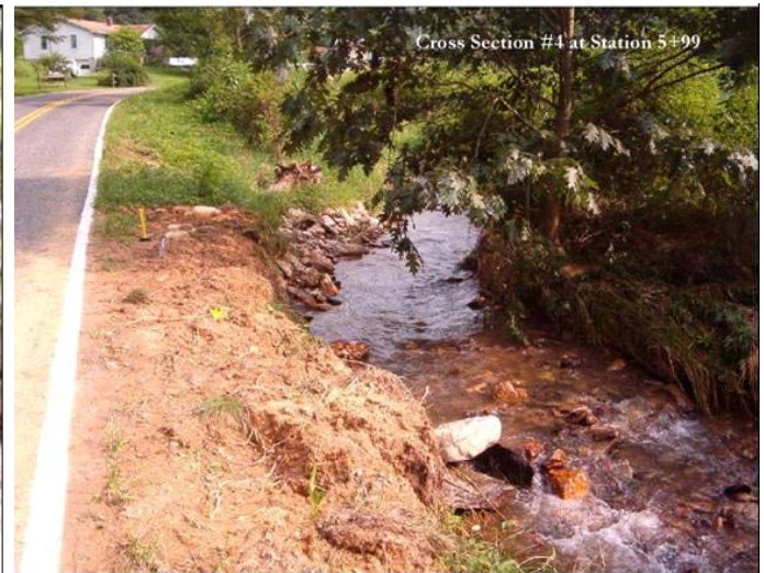
Cross-section 4, downstream to upstream, July 2003.
