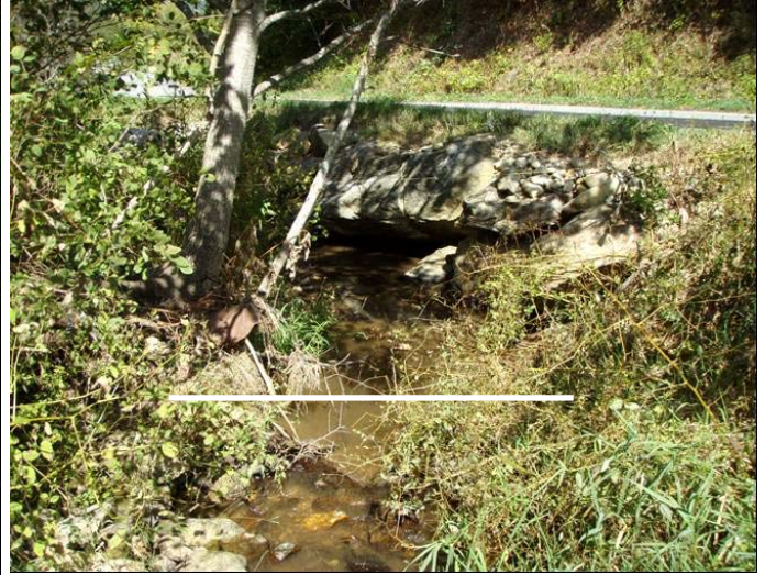
Cross-section 4, looking downstream, September 2007.
