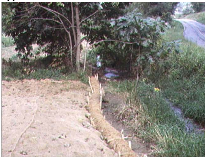
Photo sta. 5+99, looking downstream, August 1999.
