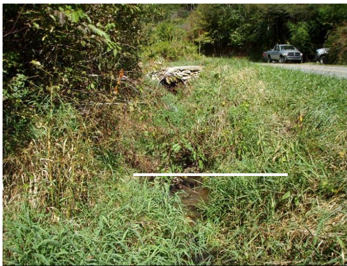
Cross-section 3, upstream to downstream, September 2007.
