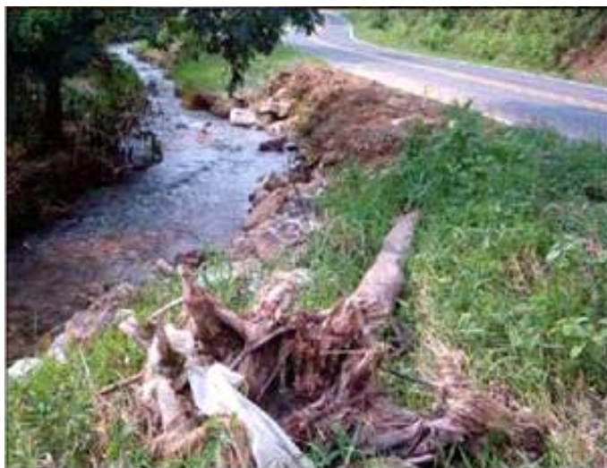
Photo sta. 5+99, looking downstream, July 2003.
