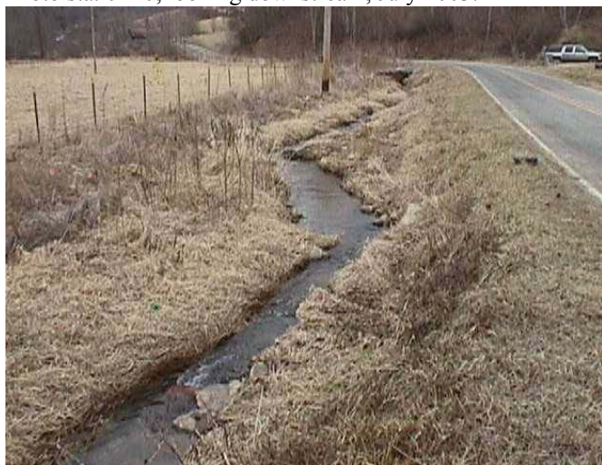
Photo sta. 2+21, looking downstream, January 2001.
