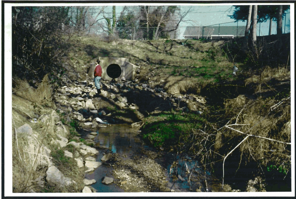
Culvert Under Lenoir Street Upstream Project Limit
