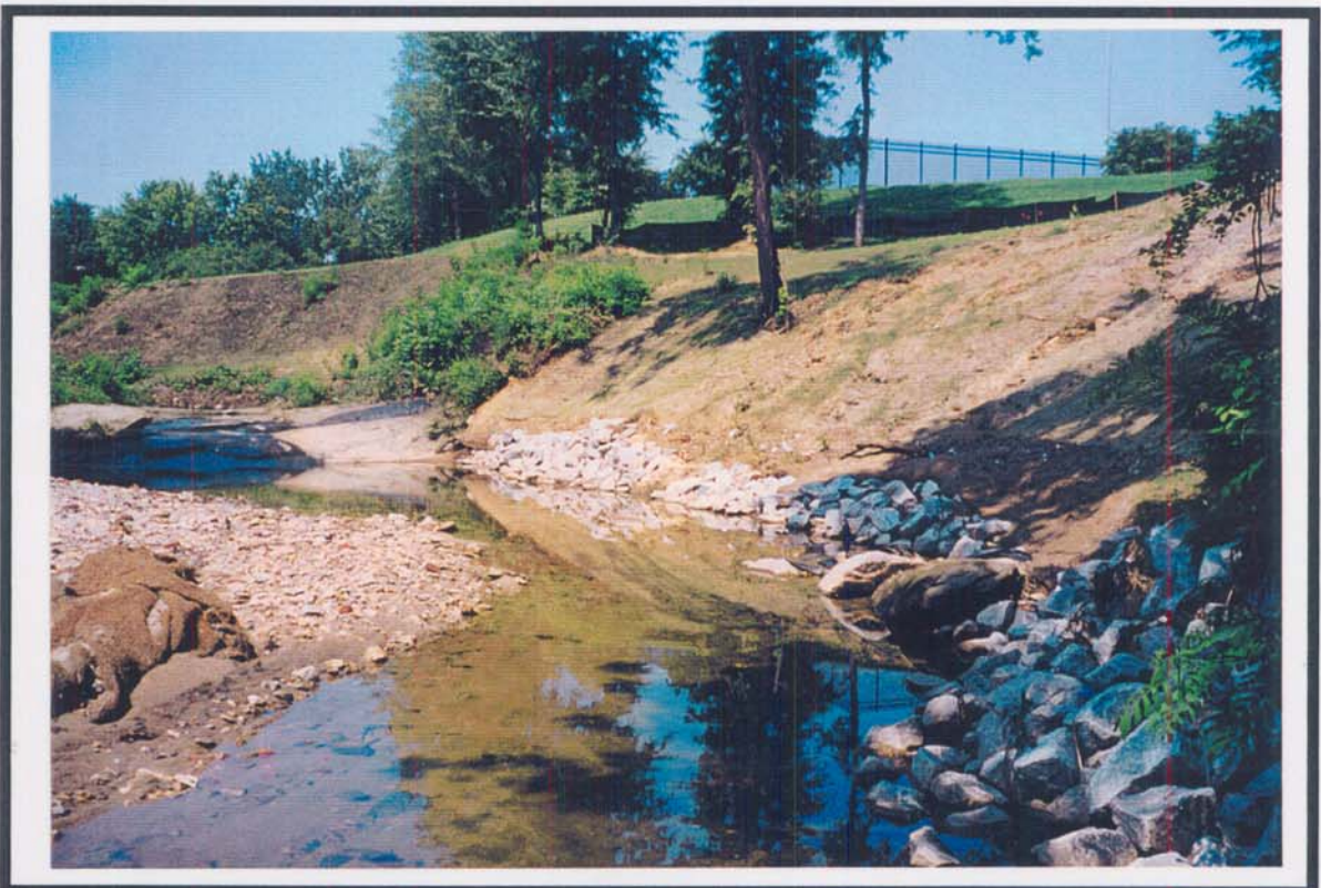
Cross Section #5 Main Channel As Viewed Looking Upstream
