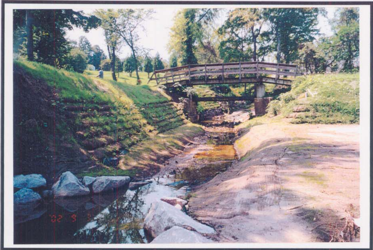
Cross Section #4 Tributary As Viewed Looking Upstream
