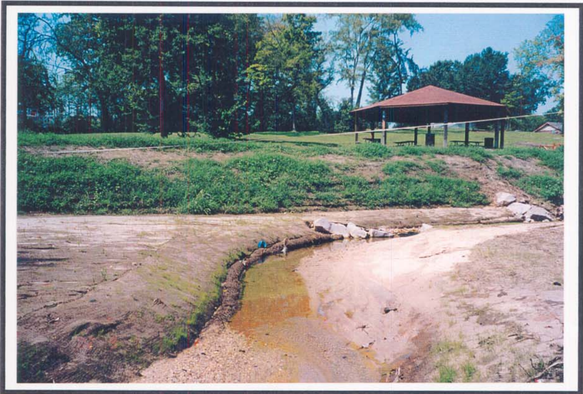
Cross Section #4 Main Channel As Viewed Looking Upstream
