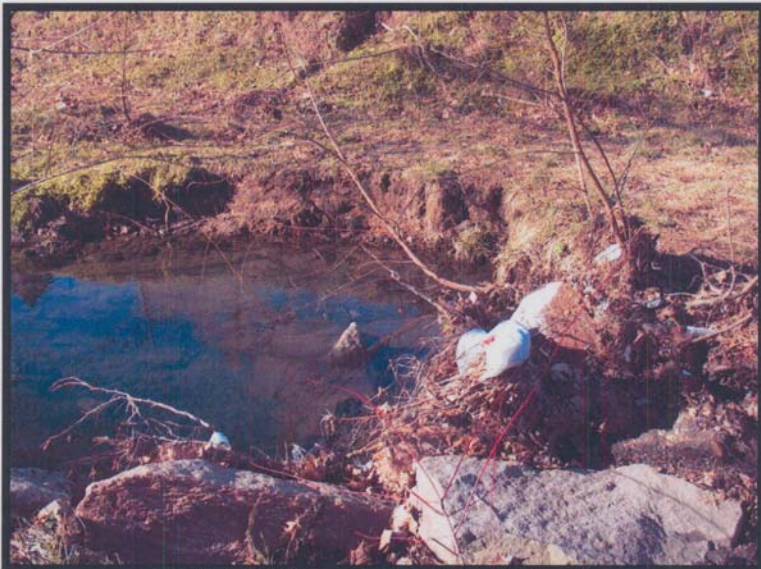
STA 4+75 Blow Out and Bank Erosion
