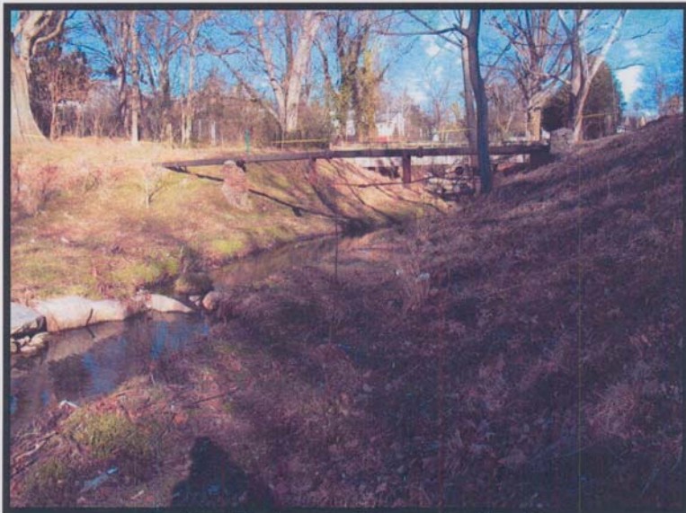
Looking Upstream at Cross Section #1
