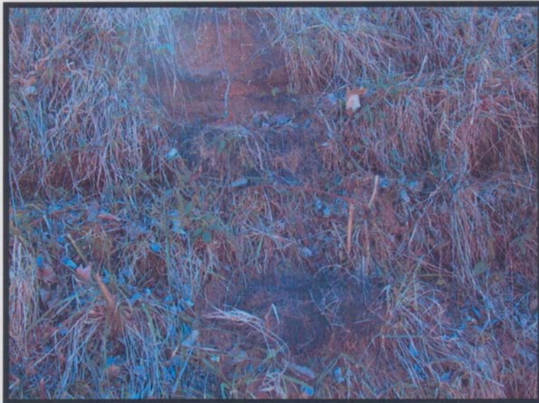
STA 15+00 GeoGrid Bank Stabilization on UT
