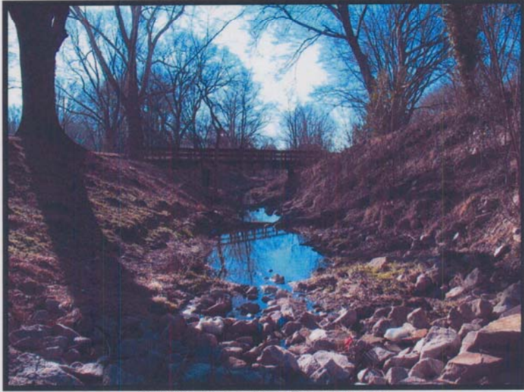
STA 0+40 Looking Downstream
