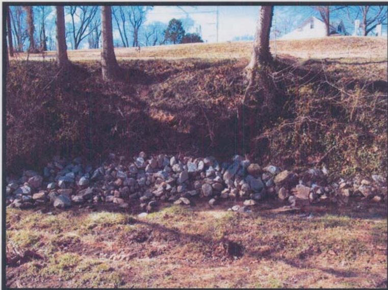
STA 11+00 Looking at Rip Rap Toe of Slope Right Bank
