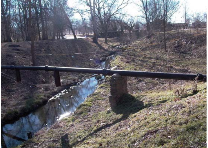
Photo of Cross-Section #1 - Looking Downstream
