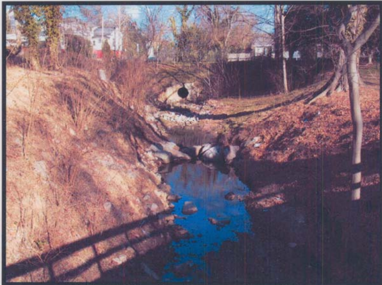
STA 1+65 Looking Upstream from Bridge
