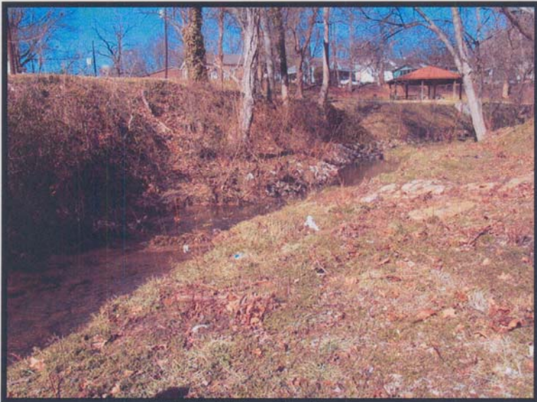
STA 11+75 Looking Upstream
