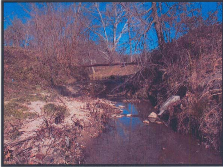
STA 13+00 Looking Upstream
