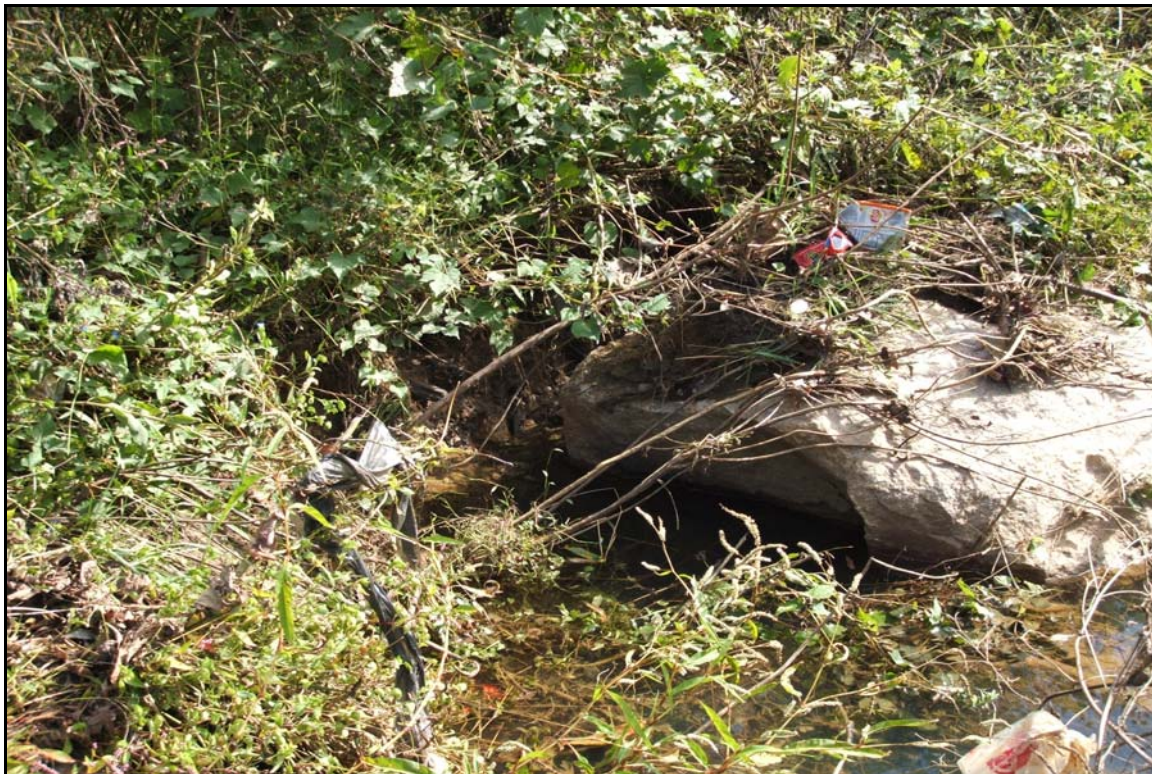
SP3 – Back arm scour on cross vane. Photo taken near station 24+90. 10/13/05 - MY 02
