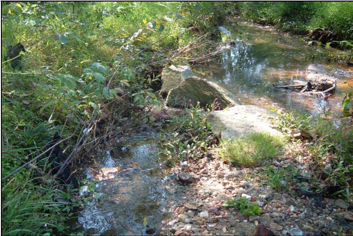
SP3 – Back arm scour on cross vane. Photo taken near station 14+50. 10/3/06 - MY 03
