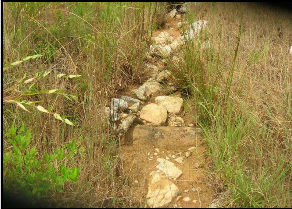
Log grade control/constructed riffle in Reach S1 (typ.)
