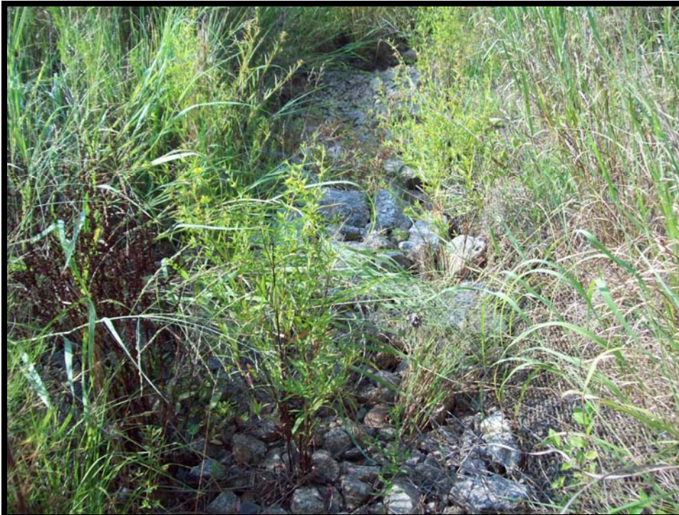
Constructed Riffle (Typ.)
