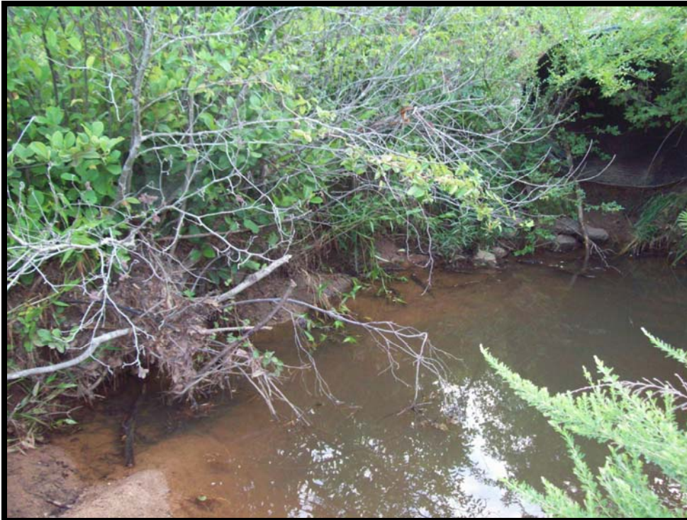
Left bank erosion @ station 10+20 facing upstream (R1)
