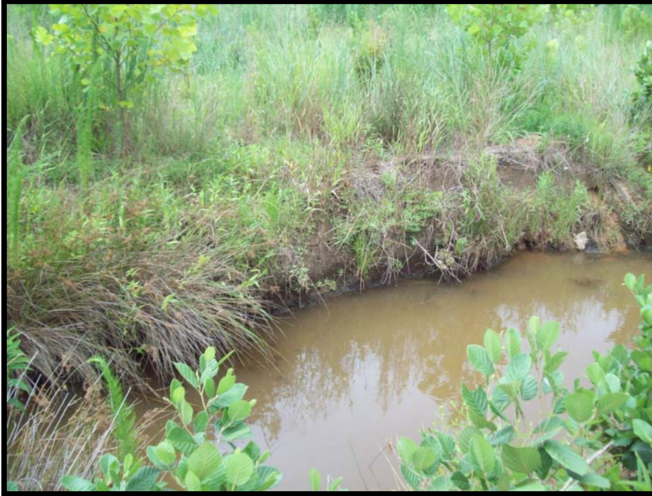
Erosion along left bank @ station 47+80 (R3)
