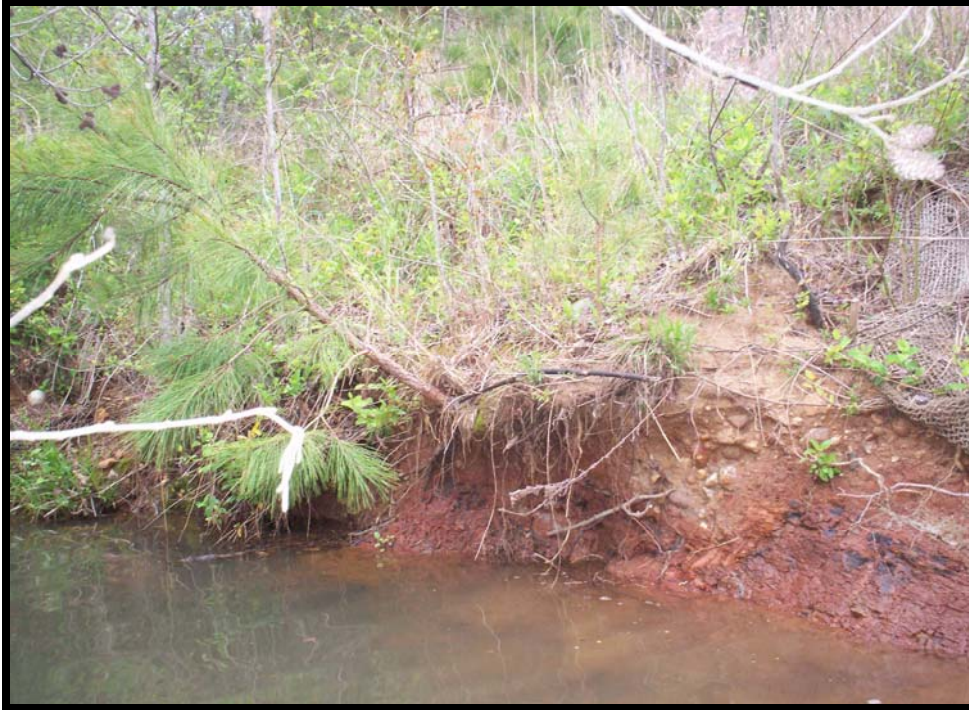
Left bank erosion @ station 10+20 facing downstream (R1)
