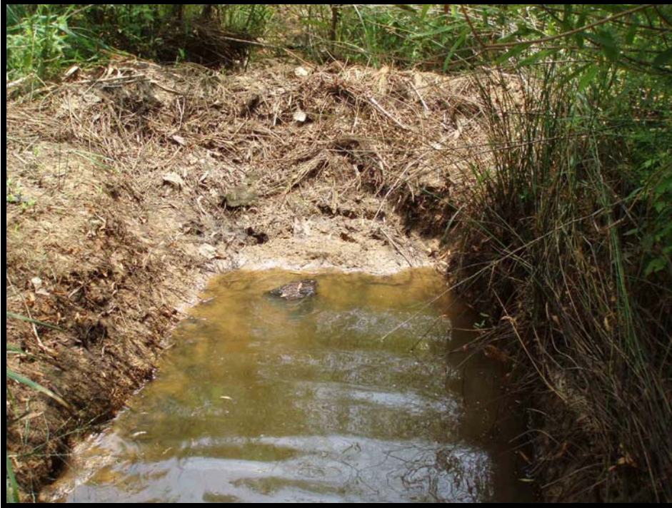
SPA5 - Beaver dam across channel @ station 33+00 (R2)
