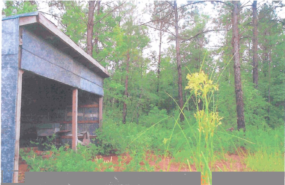
Figure 2. Mesic Pine Flatwoods behind equipment shed on center road.
