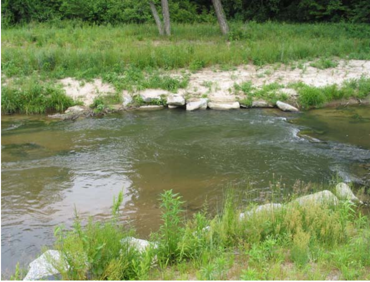
Photo 3 Cross vane at Station 1+90. Note center section shifted and piping at several locations. At high flows, the arms of the cross vane accumulate sediment and protect the banks.
