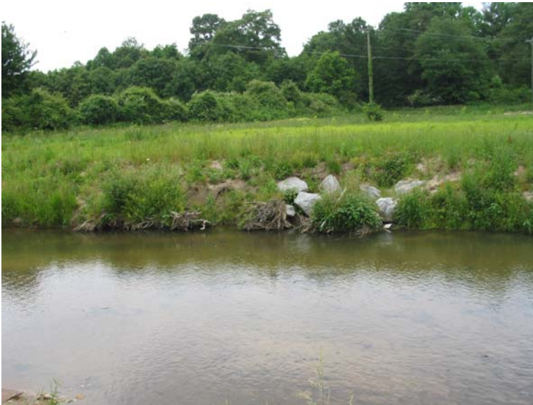
Photo 2 Pool cross-section at Station 10+50. The outside of this bend is where the most stable pool occurs other than the plunge pools below each cross vane. The low flow depth is over 5 feet just off the root wads in the bank.
