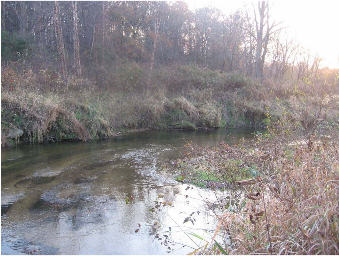
SP 5 – Looking downstream, scour of left bank
