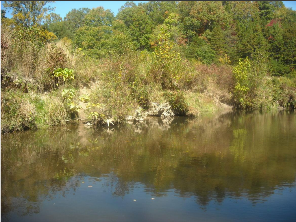
SP3: Scour behind rootwads Taken 10/13/2008
