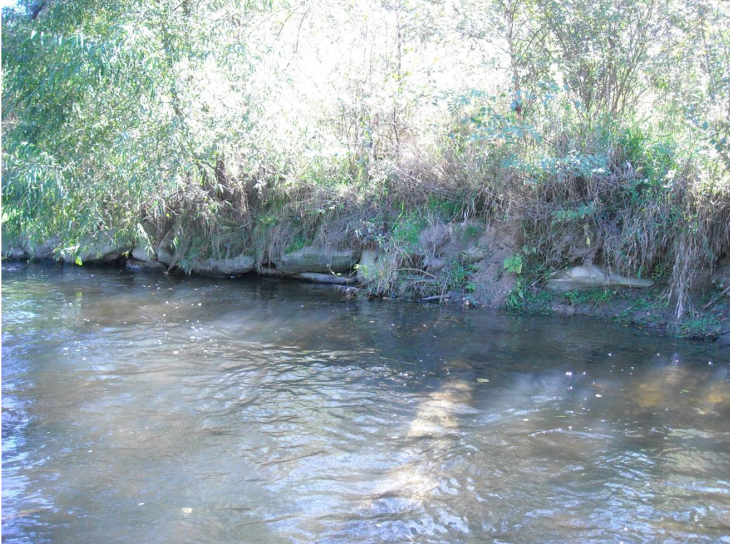
SP2: Eroding bank with undercut rootwads Taken 10/13/2008
